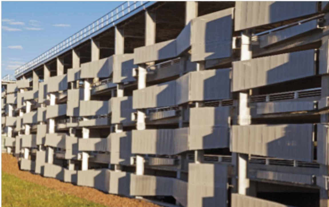
FIGURE 10: The façade design features recycled aluminum and maximizes daylight and ventilation through an open air design.
