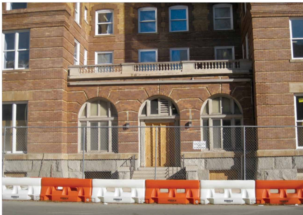
FIGURE 11. Grace Street Entrance showing rehabilitated condition, 2014. Compare with pre-construction photo above. Note paint coatings removed from stone and brick masonry at lower floors, along with restored brick masonry. Deteriorated historic wood windows have not yet been restored.
