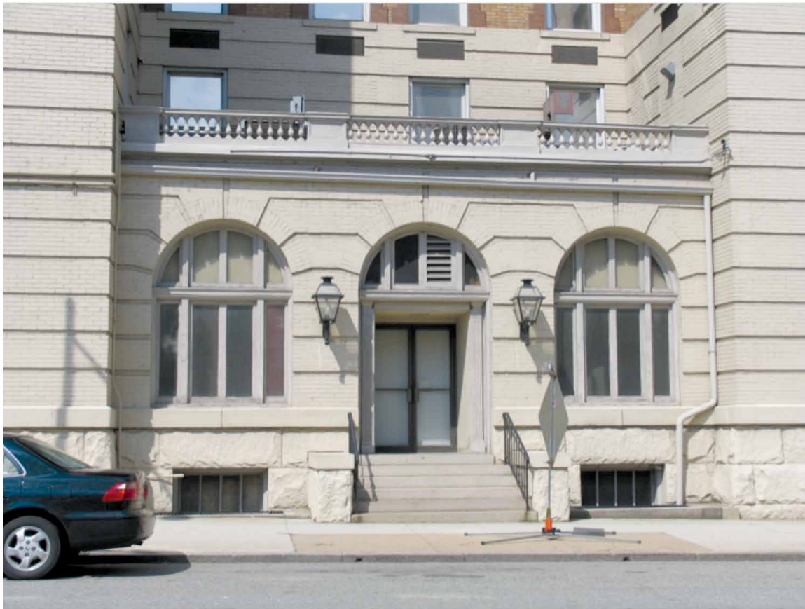
FIGURE 5. Grace Street Entrance showing Pre-Project Existing Conditions, 2006. Note painted stone and brick masonry at lower base floors and deteriorated wood and aluminum windows.
