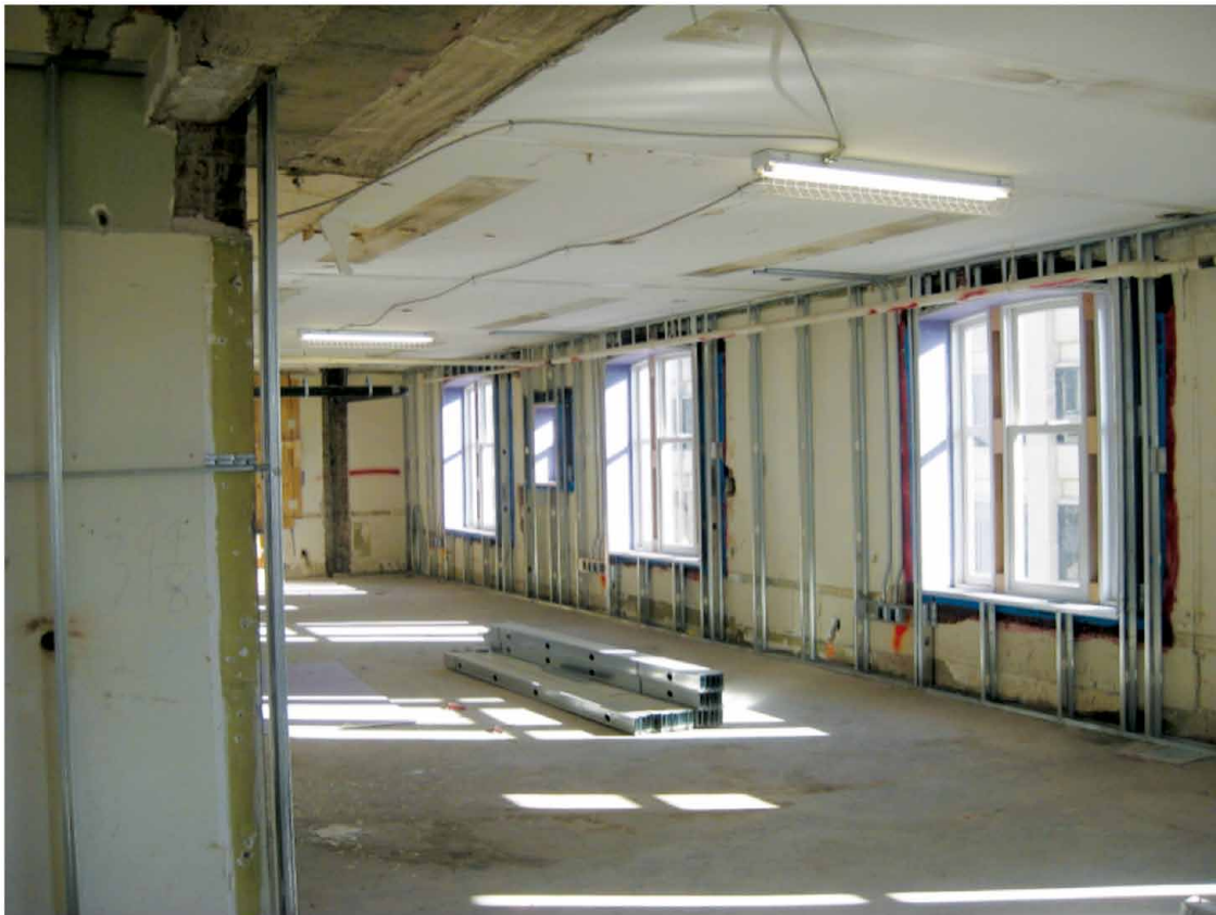
FIGURE 15. Daylight at Typical Office Floors. Full glass front walls (to be designed and built as part of the tenant interior phase) will define individual offices and the shallow floor plates will allow daylight and views to penetrate deep into the interior of the floors.
