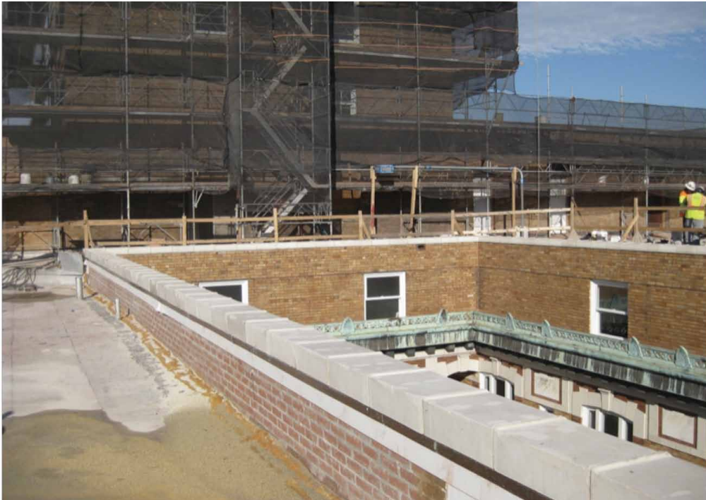
FIGURE 14. Reconstruction of masonry parapet in progress. TPO flashing is being installed in preparation for new roofing and masonry work. Note newly restored and reinstalled terra cotta capstones at right.
