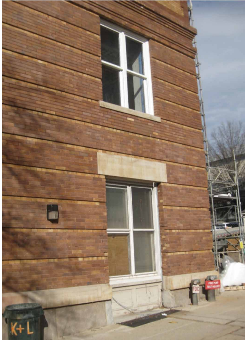
FIGURE 12. Northeast corner of the Ninth Street Façade showing restored brick and stone masonry and new replacement window at Second Floor. The First Floor window is a pre-existing deteriorated aluminum window that has yet to be replaced. The light fixture on the wall is a temporary construction fixture.
