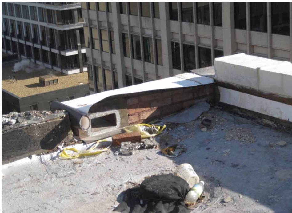
FIGURE 14. Reconstruction of masonry parapet in progress. TPO flashing is being installed in preparation for new roofing and masonry work. Note newly restored and reinstalled terra cotta capstones at right.
