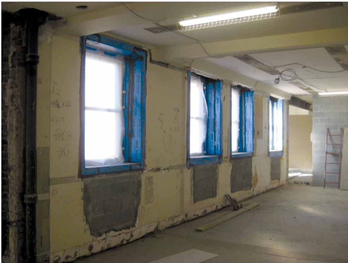
FIGURE 9. Repair of existing exterior enclosure work in progress. Note CMU infill at former through-wall HVAC unit locations, installation of new replacement insulated window units and associated window flashings, and water barrier.
