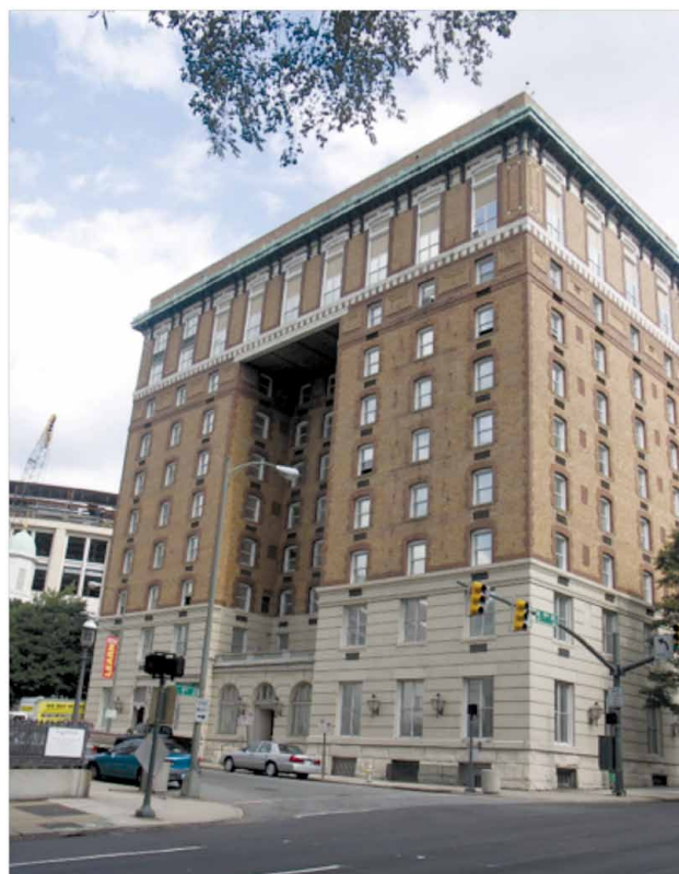
FIGURE 4. Ninth & Grace Street Corner showing Pre-Project Existing Conditions, 2006. Note painted stone and brick masonry base floors and through-wall fan coil units under deteriorated aluminum replacement windows.
