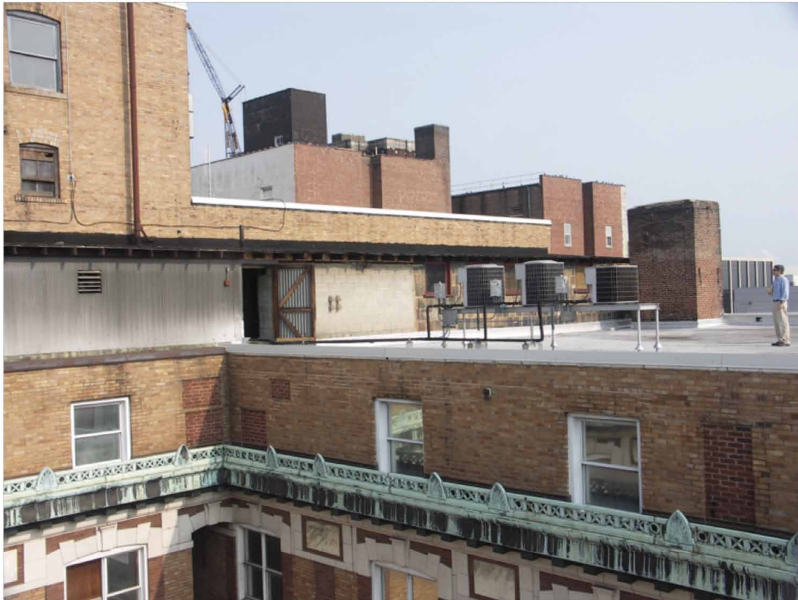
FIGURE 6. Ninth Street Courtyard Upper Floors and Rooftop showing Pre-Project Existing Conditions, 2006. Note deteriorated brick masonry joints, mismatched masonry infill, outdated rooftop mechanical equipment, deteriorated aluminum replacement windows, and incompatible rooftop structures to be removed.
