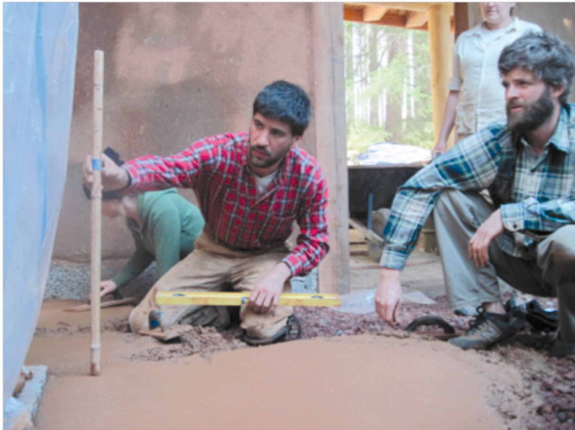
FIGURE 18. Installing an earthen floor during an Aprovecho workshop.
