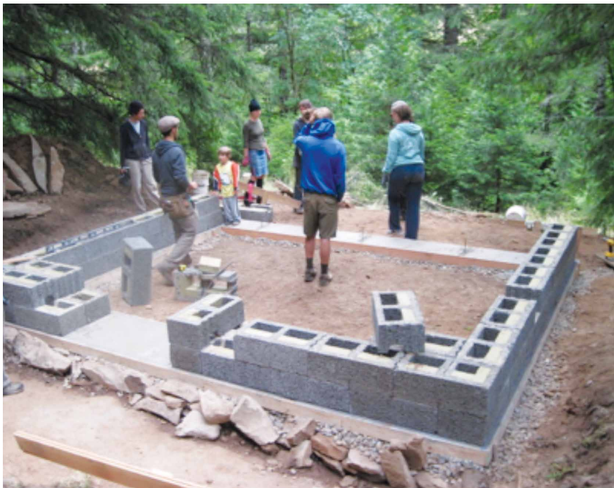
FIGURE 9. "Faswall" blocks being placed on top of a 4" bond beam.
