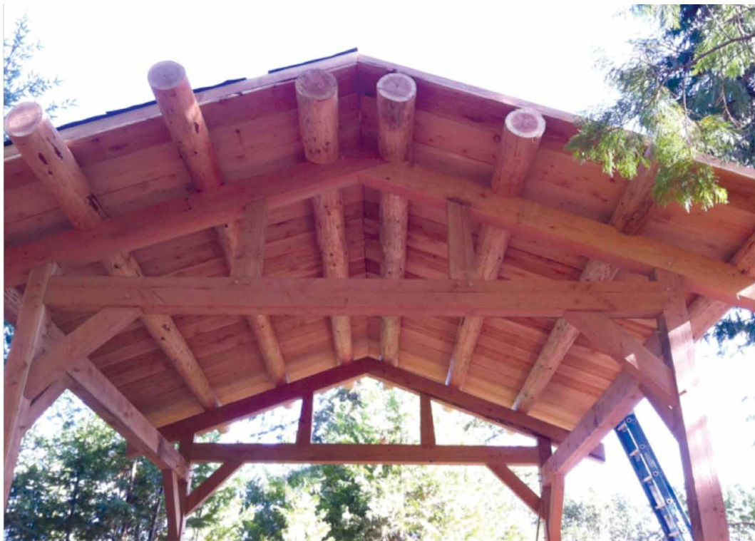
FIGURE 13. Roundpole purlins on top of timber frame.
