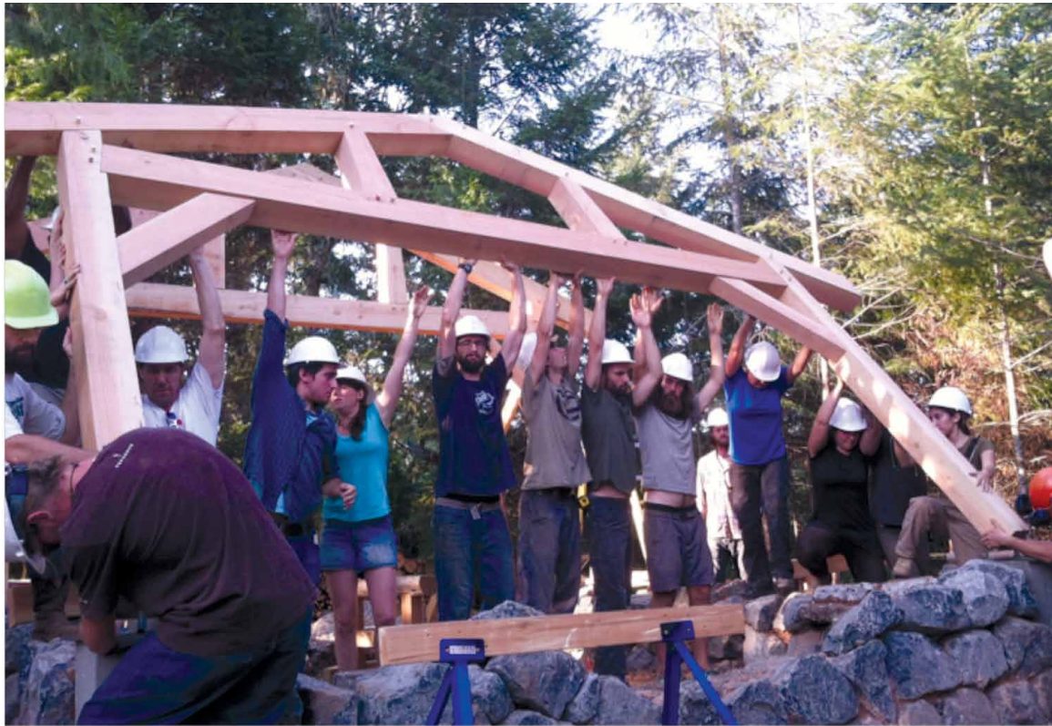
FIGURE 12. Timber frame raising during 2014 Shelter Series.
