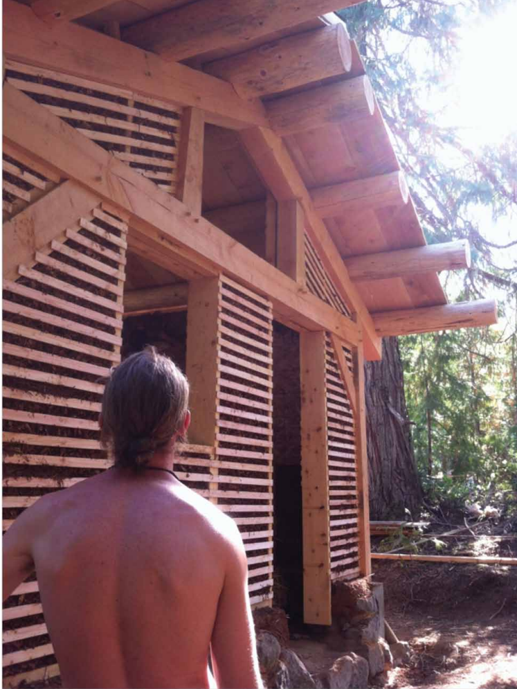
FIGURE 17. A slip and chip wall before plaster. The clay covered wood chips fill the cavities defined by the wooden lathe and provide insulation.
