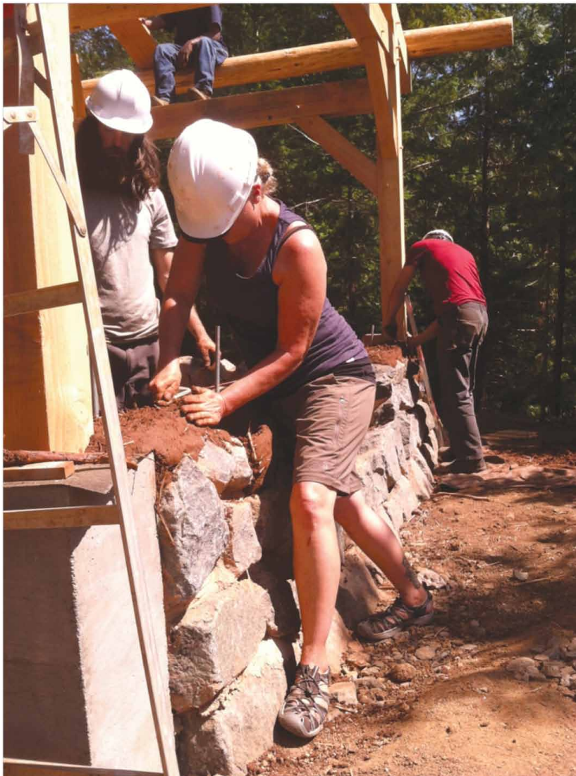
FIGURE 21. Applying a cob bond beam to a stone stem wall.
