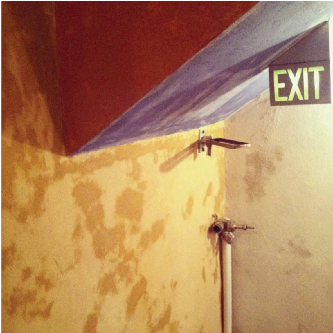
FIGURE 20. Four different clay paints drying during a retrofit of a historic downtown Cottage Grove building. The lighter colors are the finished colors.
