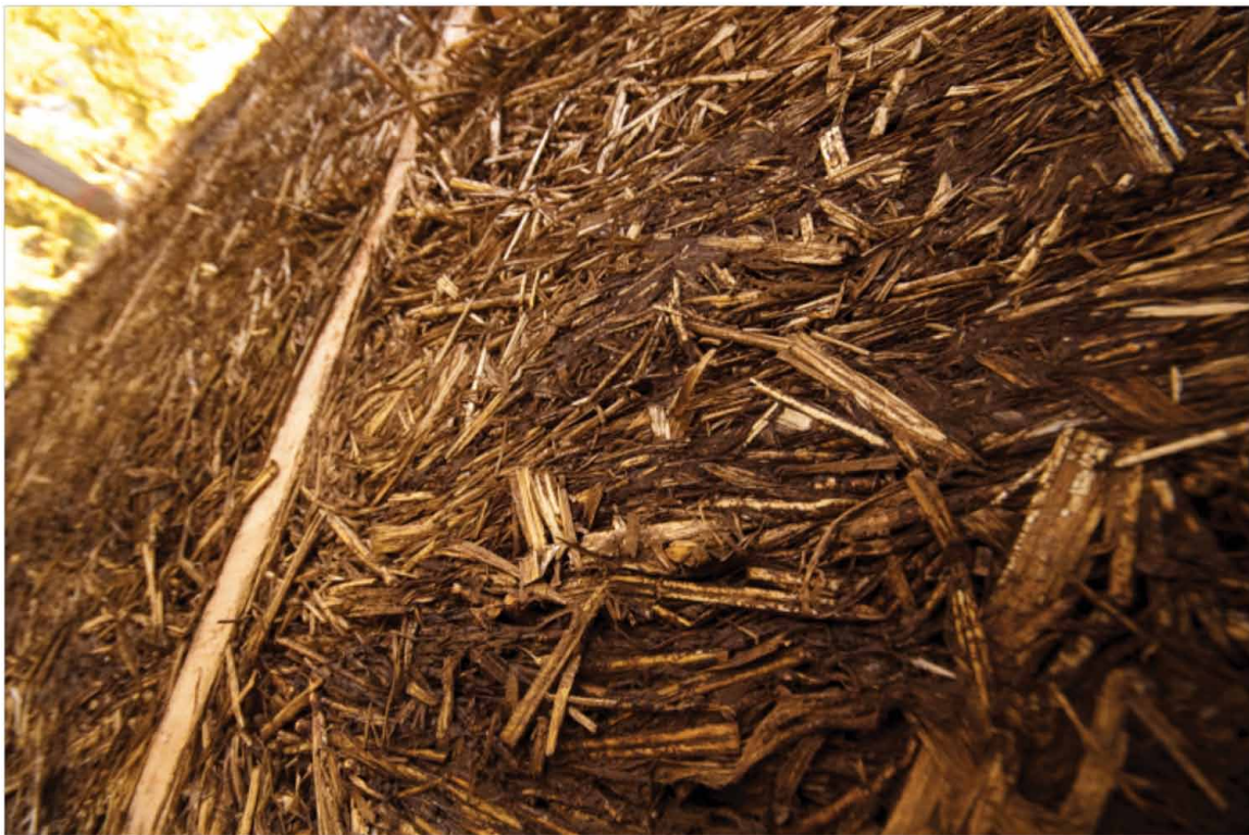
FIGURE 16. Up close photo of a LCS wall which is a mix of clay and straw packed in between larsen trusses.
