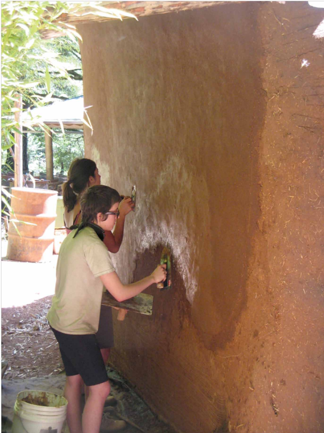
FIGURE 19. Students applying a smooth clay finish plaster on top of a rough base plaster.
