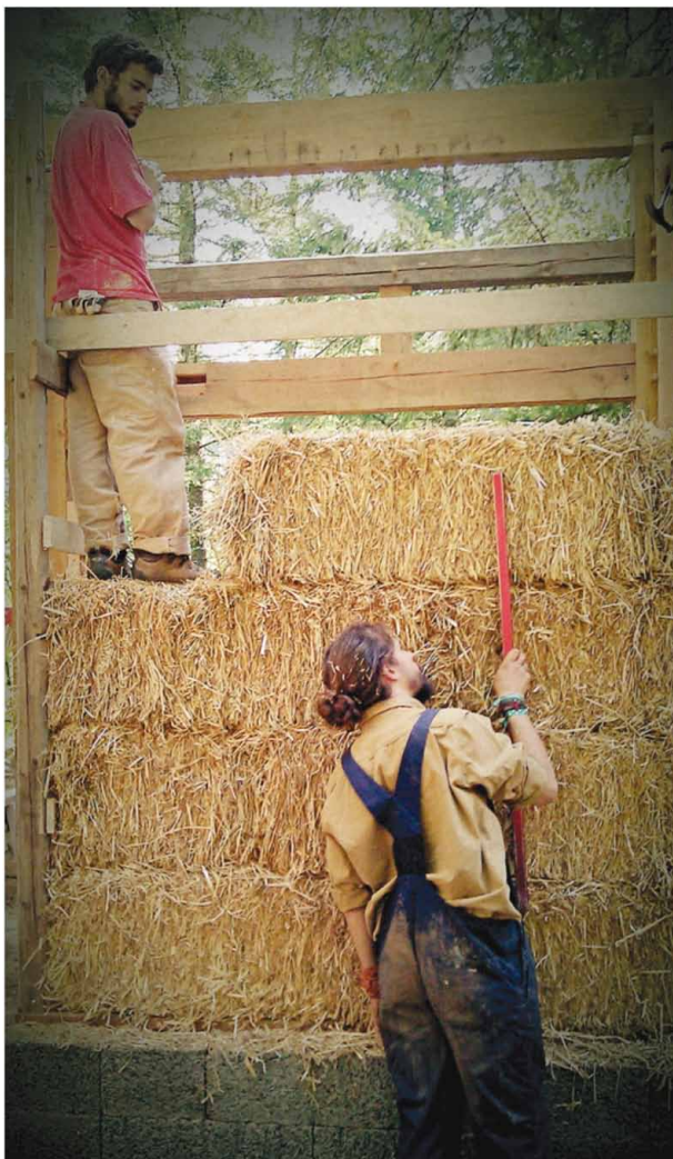
FIGURE 15. A student ensuring a strawbale wall remains plumb before pinning with bamboo stakes.
