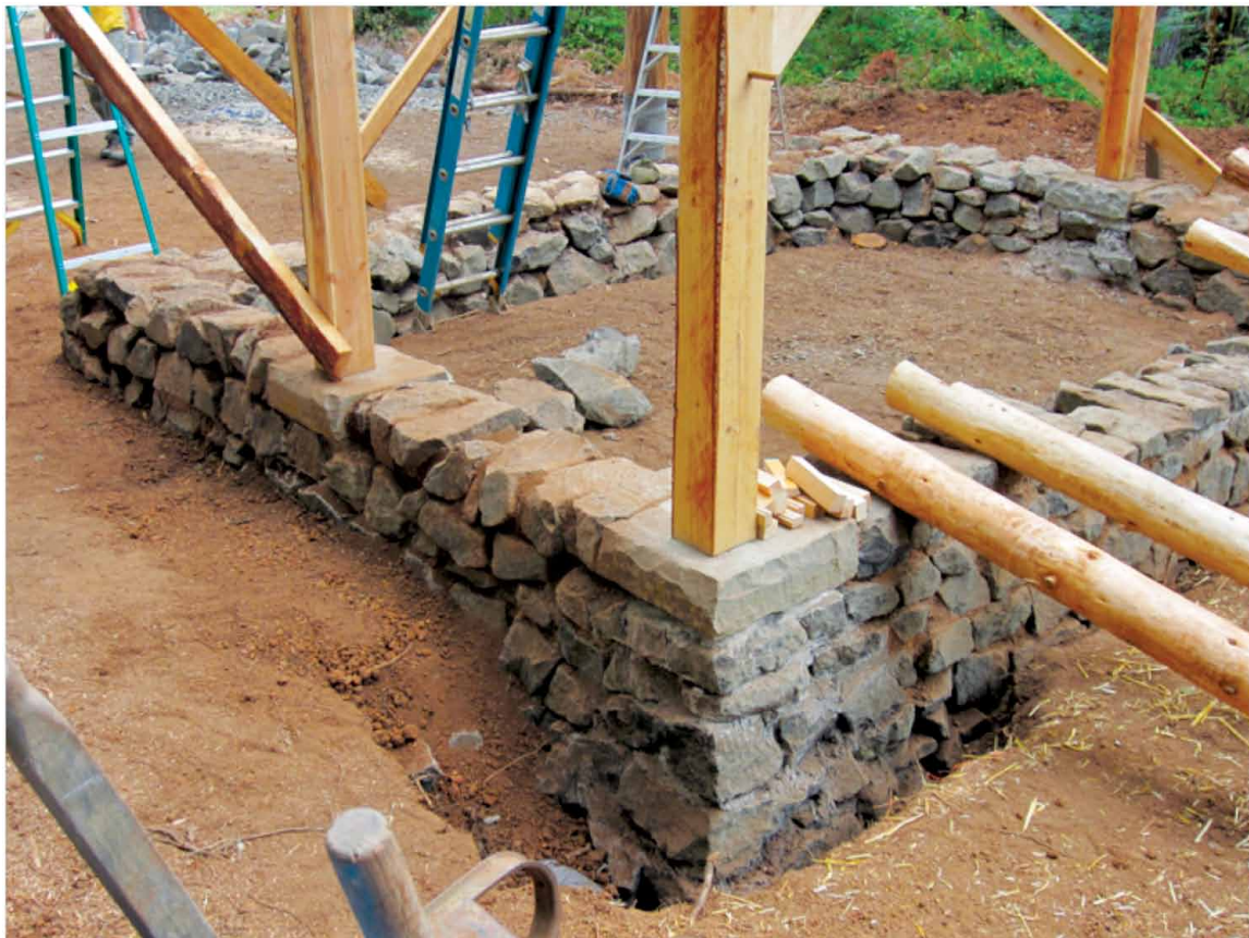
FIGURE 11. Stone foundation made mostly from local basalt.
