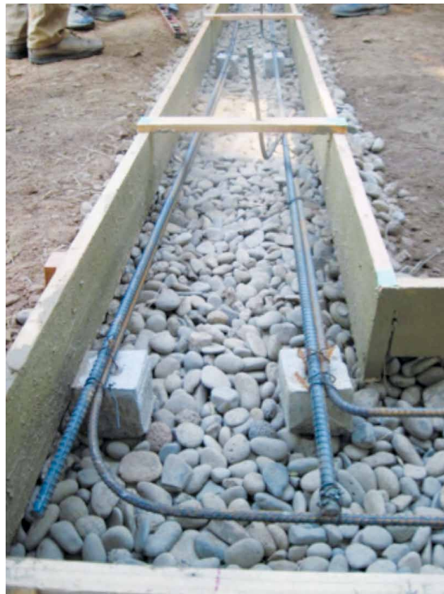
FIGURE 8. Form to receive a concrete bond beam placed on top of a rubble trench.
