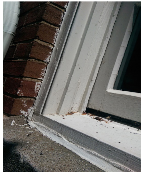
FIGURE 4. Single paned window with ledge.
