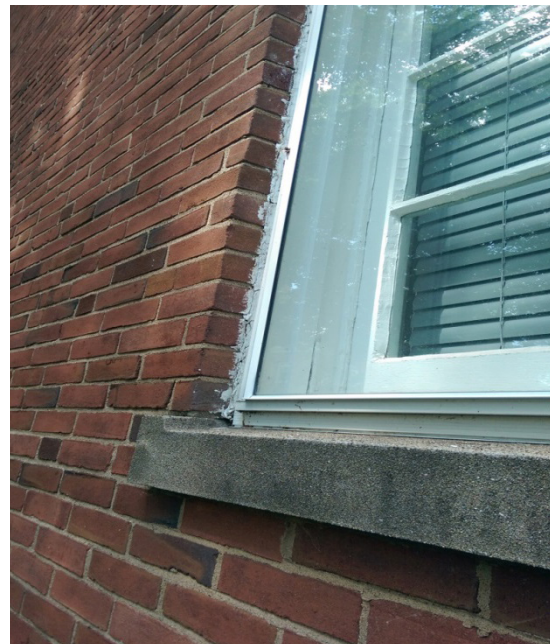
FIGURE 5. Storm Window.
