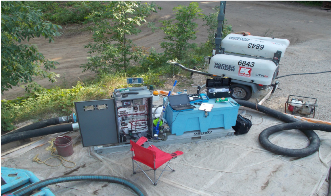
FIGURE 5. Automated dewatering systems are an excellent way to manage risk; however, remember manual oversight and verification are also needed to ensure compliance.
