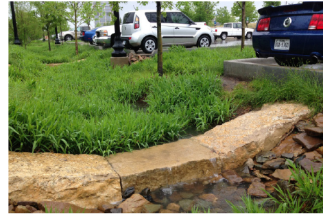
FIGURE 10. Pavement runoff at the north visitor parking lot flows to bioswales where grasses, sedges, and stone check dams cleanse the water before it is piped and released into the park's drainage features.
