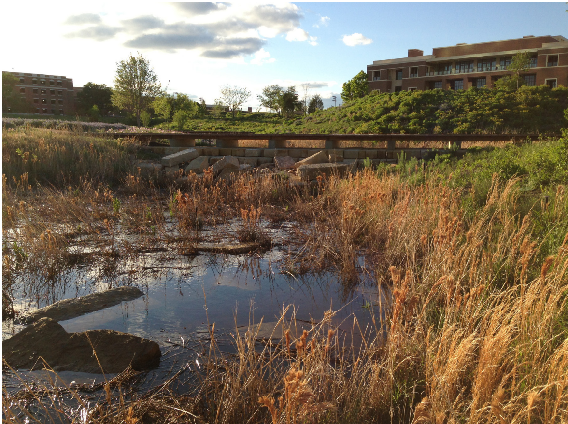
FIGURE 12. The east and west Bioswales spill into the Wet Prairie where water slowly percolates into the 252,000 gallon irrigation tank below it.
