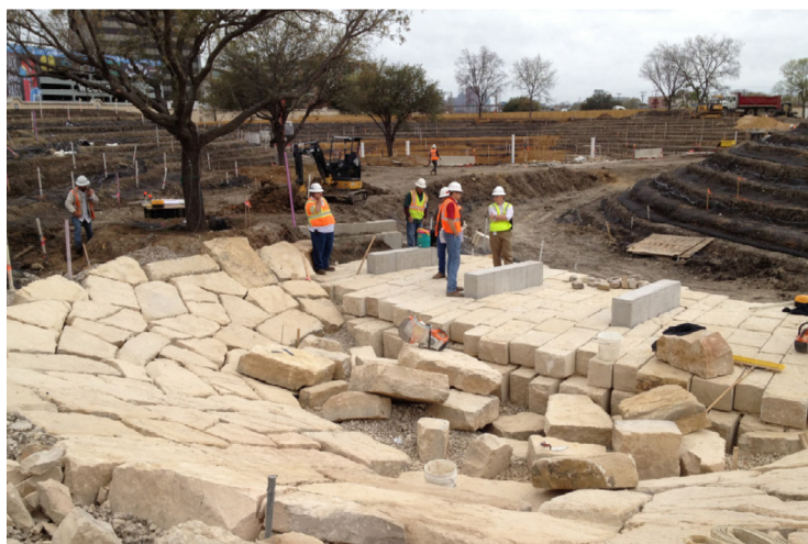
FIGURE 17. Limestone slabs line the forebay to reduce the erosive forces of downpours. Random stones at the mouth of the forebay disperse water velocity.
