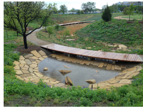
FIGURE 11. Water from upland parking is piped to the stone forebay where it can settle and be slowly released through 2" wide joints in the stone block ford below the bridge.
