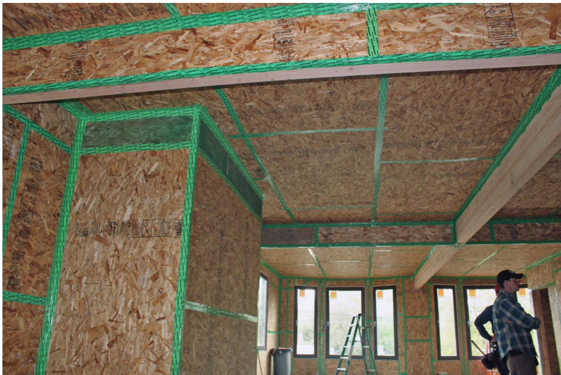
FIGURE 7. Air barrier created by OSB panels taped with vapor permeable Siga tape.
