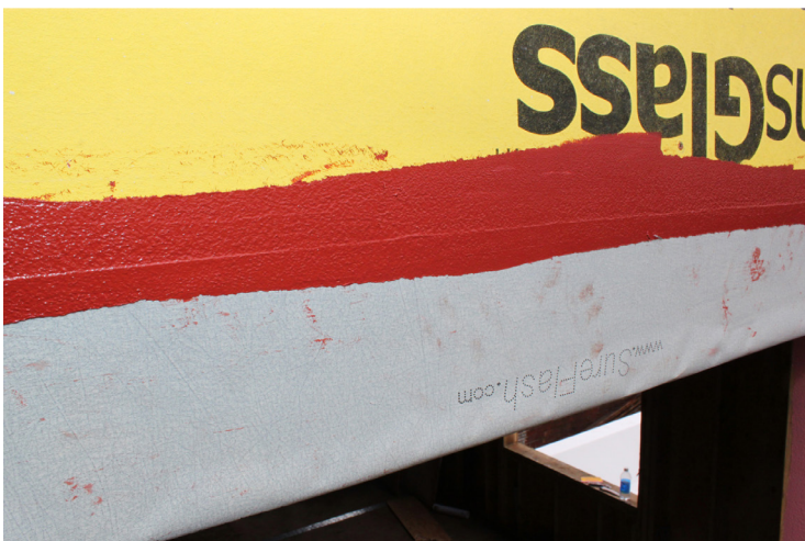
FIGURE 11. Liquid applied flashing extended pas the SureFlash membrane at least nine inches out from rough opening.
