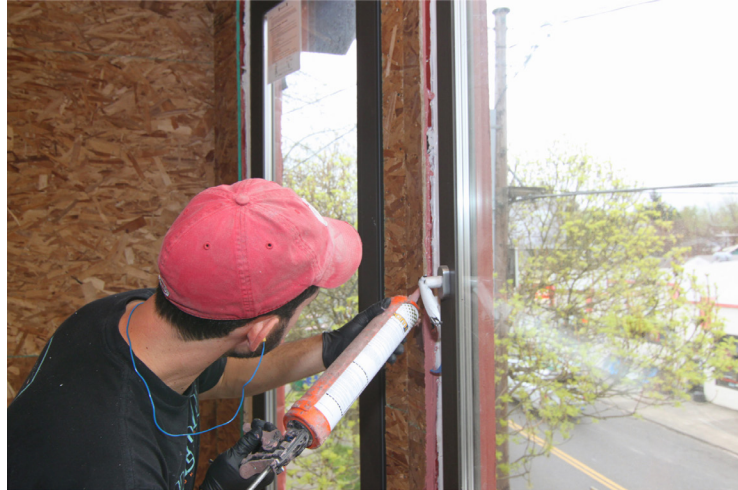
FIGURE 12. Air Dam sealant being applied.
