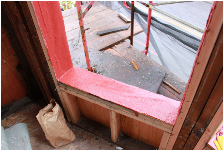
FIGURE 10. Liquid applied flashing applied to rough opening.
