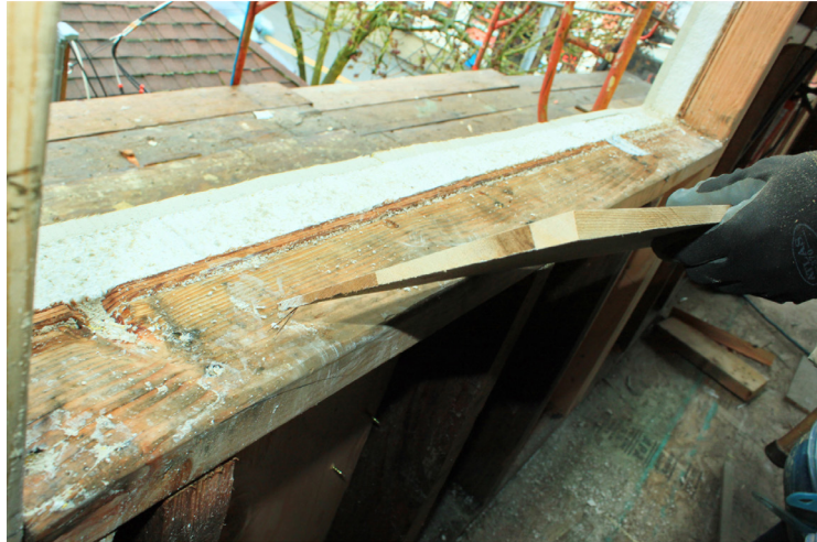
FIGURE 8. Secondary sill being placed to span the framed sill, exterior EPS, and cladding layers.
