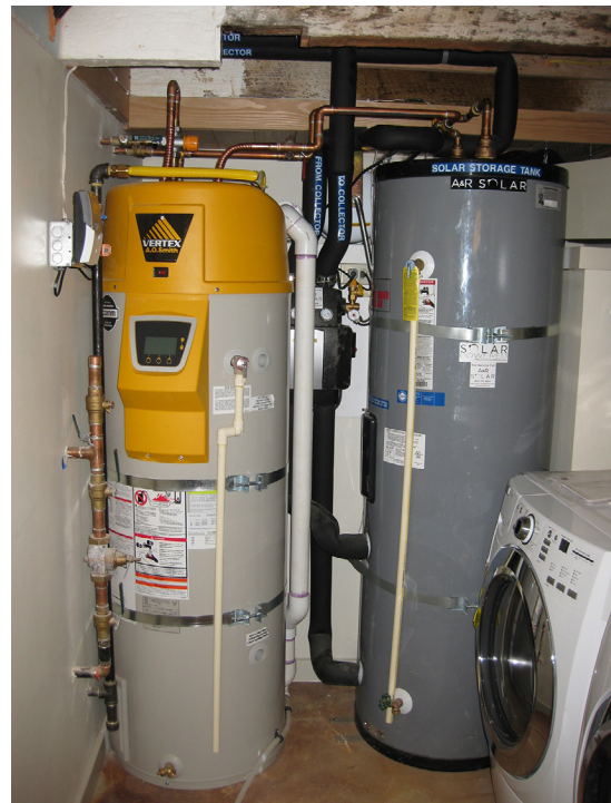
Solar Hot Water Storage paired with AO Smith Vertex Hot Water Tank.
