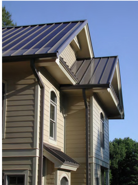
FIGURE 6. Custom gutters and downspouts for each home. We have observed the collection of condensate during the summer months when we have had no rain fall. ©2014 CCLLC, Cadmus Construction LLC, Roswell, GA 30075.
