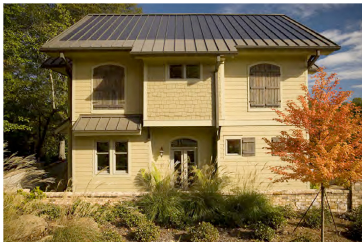
FIGURE 14. Southern Facing Elevation features: integrated solar pv & thermal system, deep overhangs and cantilevers that are strategically placed to act as solar shading devices. ©2014 CCLLC, Cadmus Construction LLC, Roswell, GA 30075.
