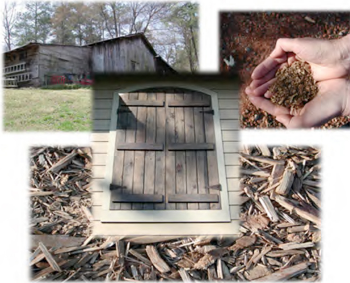
FIGURE 13. Old barn prior to deconstruction; sawdust from planing barn wood [used as ground cover for solar staging area]; barn wood shutters; wood chips [used for site stabilization]. ©2014 CCLLC, Cadmus Construction LLC, Roswell, GA 30075.
