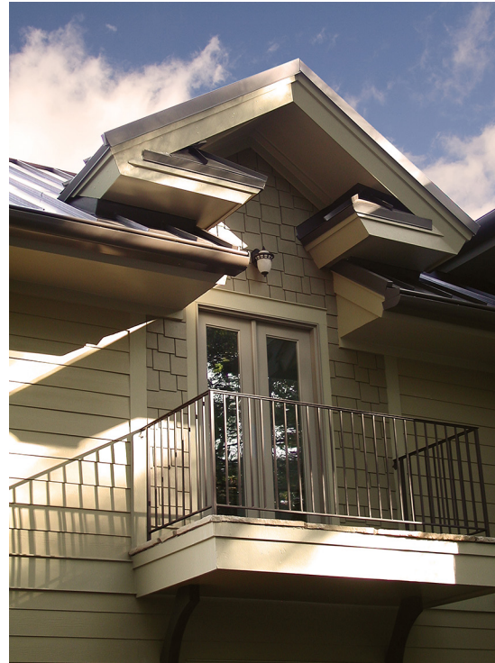
FIGURE 15. Deep overhangs and balcony [used as a solar shading device]. ©2014 CCLLC, Cadmus Construction LLC, Roswell, GA 30075.
