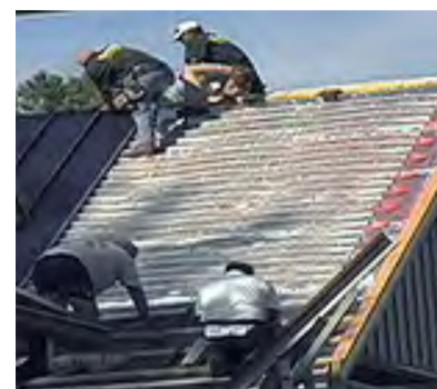
FIGURE 16. Installing the building integrated solar photovoltaic and solar thermal system. ©2014 CCLLC, Cadmus Construction LLC, Roswell, GA 30075.
