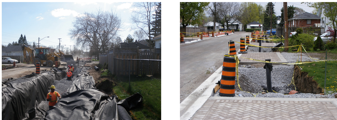
FIGURE 12. Schematic of the bioswale with the perforated pipe system and the permeable paver driveways at the Lakeview “green street” retrofit project.
