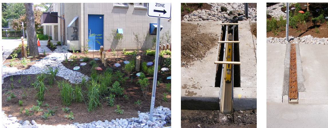
FIGURE 18. Rock channel lined with an impermeable liner (L), grate inlet retrofitted into the existing sidewalk (center), and overflow/outlet grate (R).
