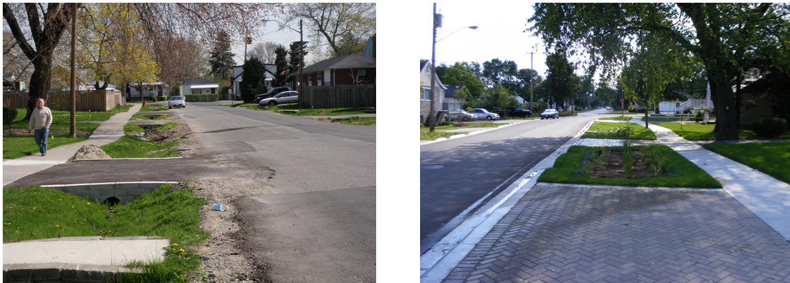
FIGURE 9. Third Street, Mississauga, ON. Before (L): ditched system had poor conveyance, failing headwalls, standing water, and poor aesthetics. After (R): bioswales and permeable pavement driveways provide improved water quality and aesthetics.
