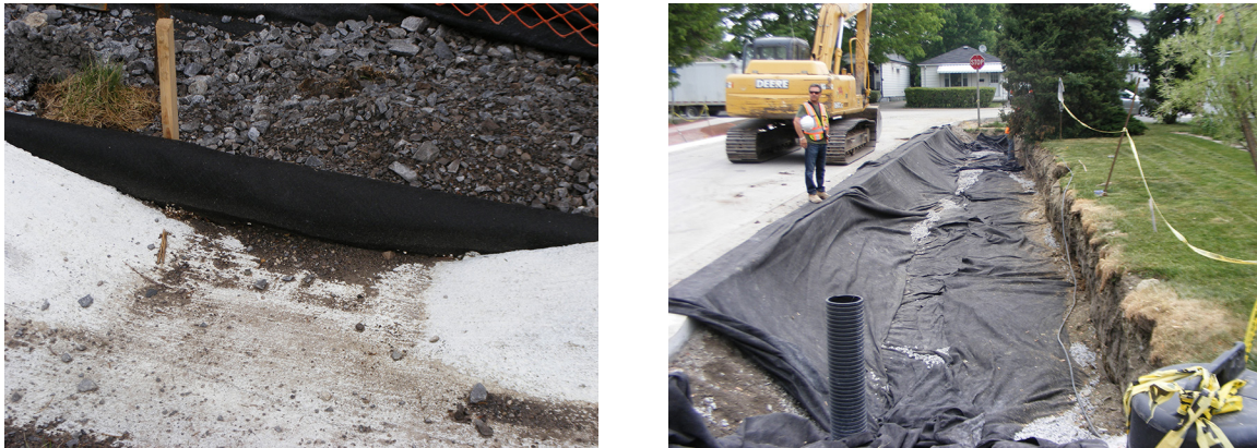
FIGURE 13. Inlet sediment barrier protects from sediment contamination prior to media placement (R) and sacrificial geotextiles area used to protect the granular material from slumping and atmospheric deposition of construction sediment.
