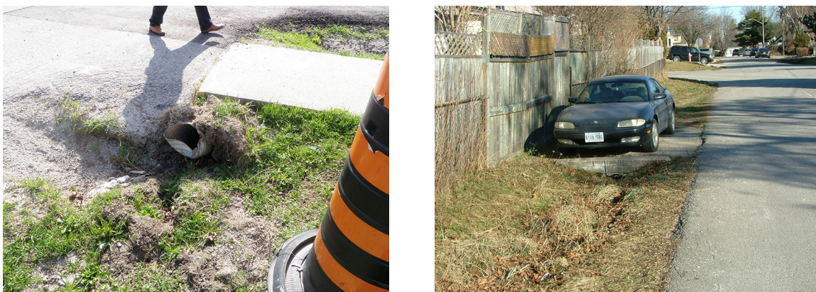
FIGURE 10. Failed culvert and unapproved parking encroaches on the municipal ROW and blocks drainage.
