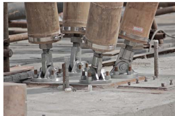
FIGURE 7. Concrete-filled bamboo culms with bolts and clamps. (a) roof level (b) foundation level (photos used with permission from MUDI architects, Shanghai).
