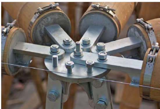
FIGURE 7. Concrete-filled bamboo culms with bolts and clamps. (a) roof level (b) foundation level (photos used with permission from MUDI architects, Shanghai).
