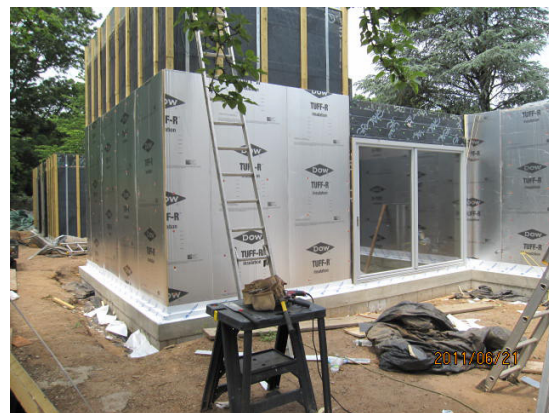
Exterior insulation being installed after windows and doors.
