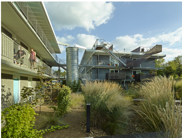
FIGURE 4. Rain garden with galvanized culvert cistern used to capture storm water from roof.
