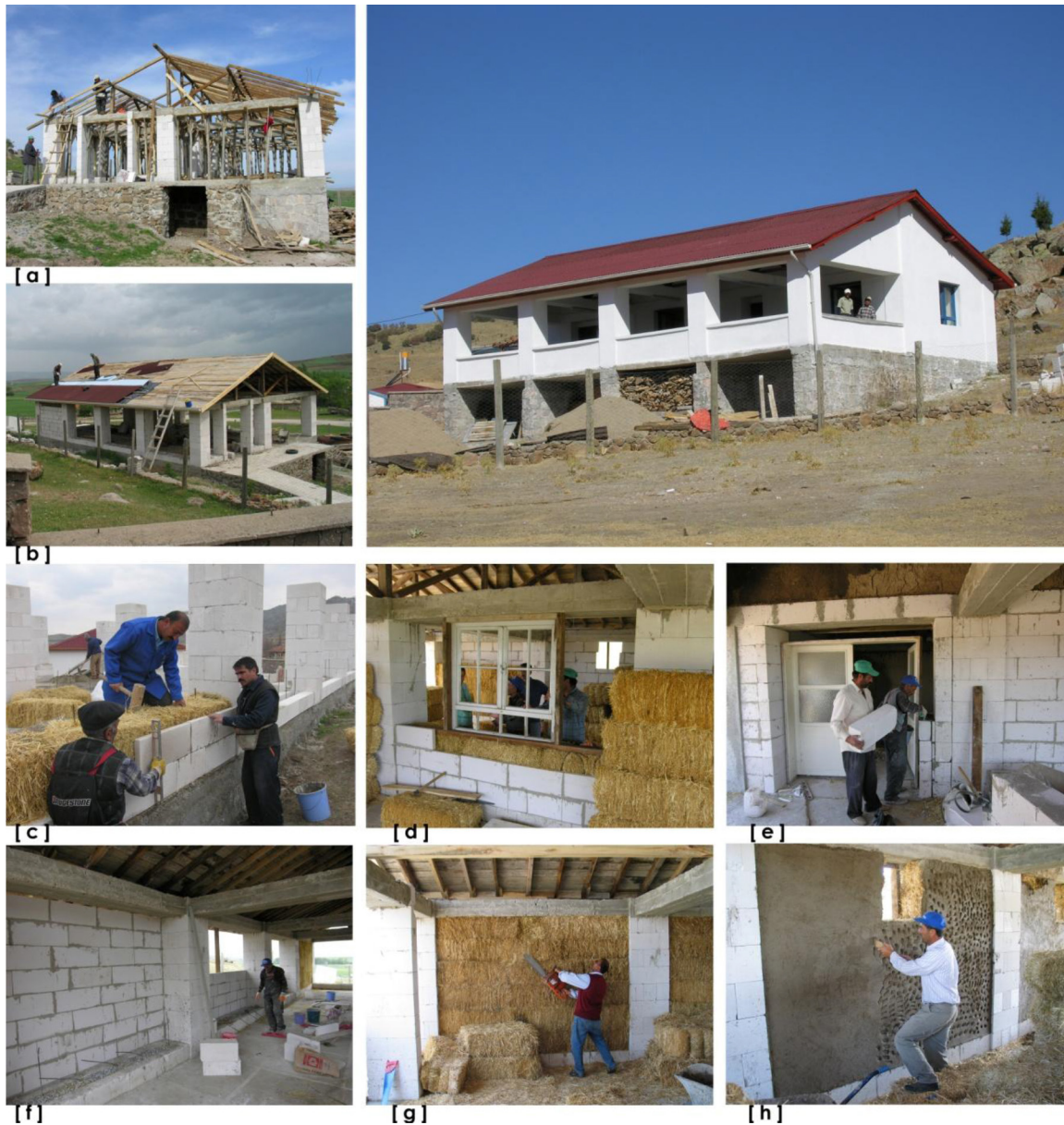
FIGURE 5. The Strawbale Conservation Workshop: [a] timber roof structure, concrete lintels and AAC piers on stone foundations; [b] laying layers of insulation on the roof; [c] wall composed of strawbales and AAC blocks; [d] installing a re-used door; [e] installing a re-used door; [f] interior view of external layer of AAC blocks; [g] trimming the straw bales; [h] plastering interior wall surface with mud and straw mixture.
