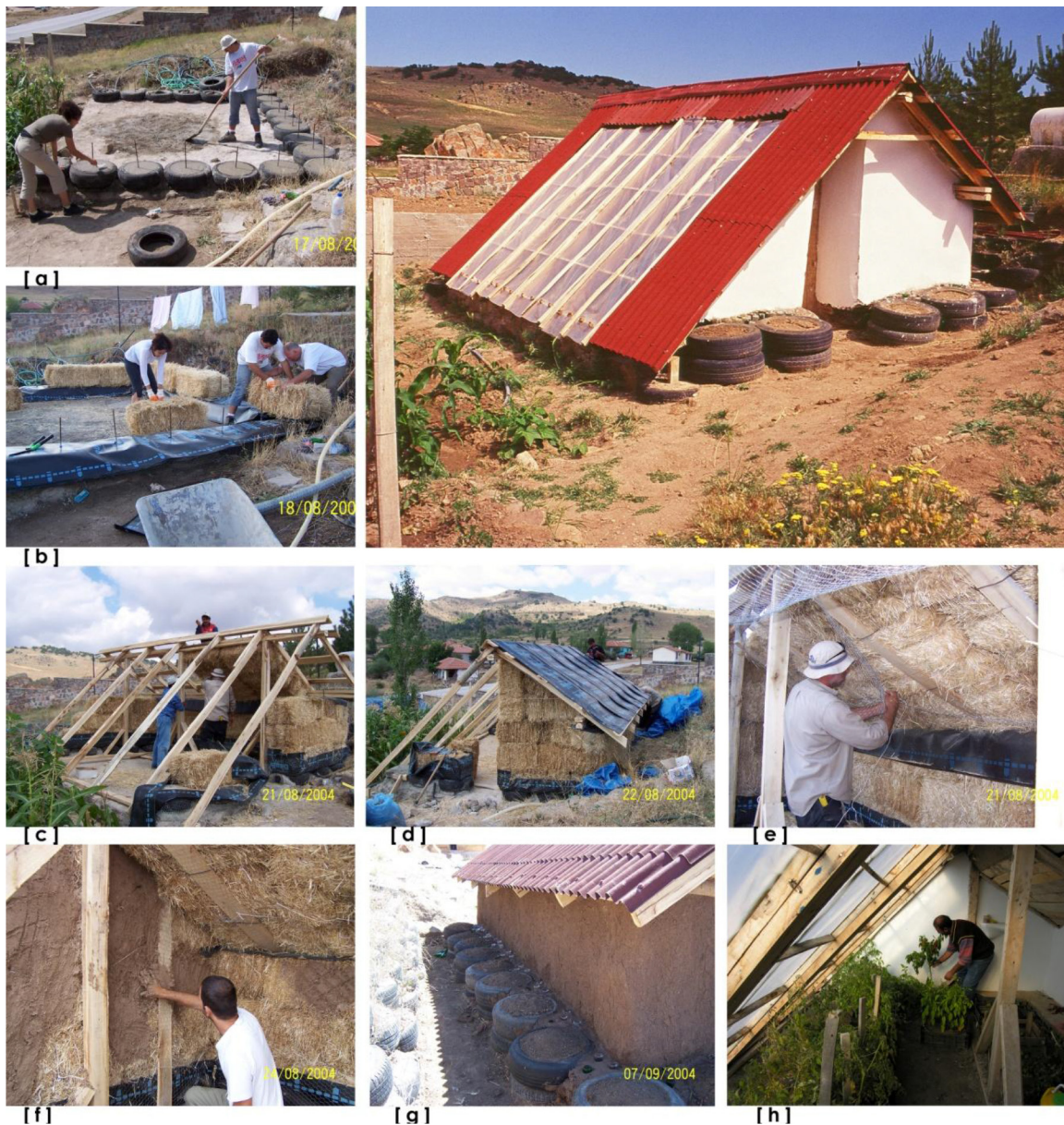
FIGURE 1. The Strawbale Greenhouse: [a] laying the foundations; [b] anchoring the first row of strawbales for the walls; [c] erecting the wooden structure; [d] roof insulation; [e] sewing on the chicken-wire before mud-rendering; [f] plastering the bales with mud and straw mixture; [g] plinth protection made of old tires, bottles and mud; [h] interior of the greenhouse.
