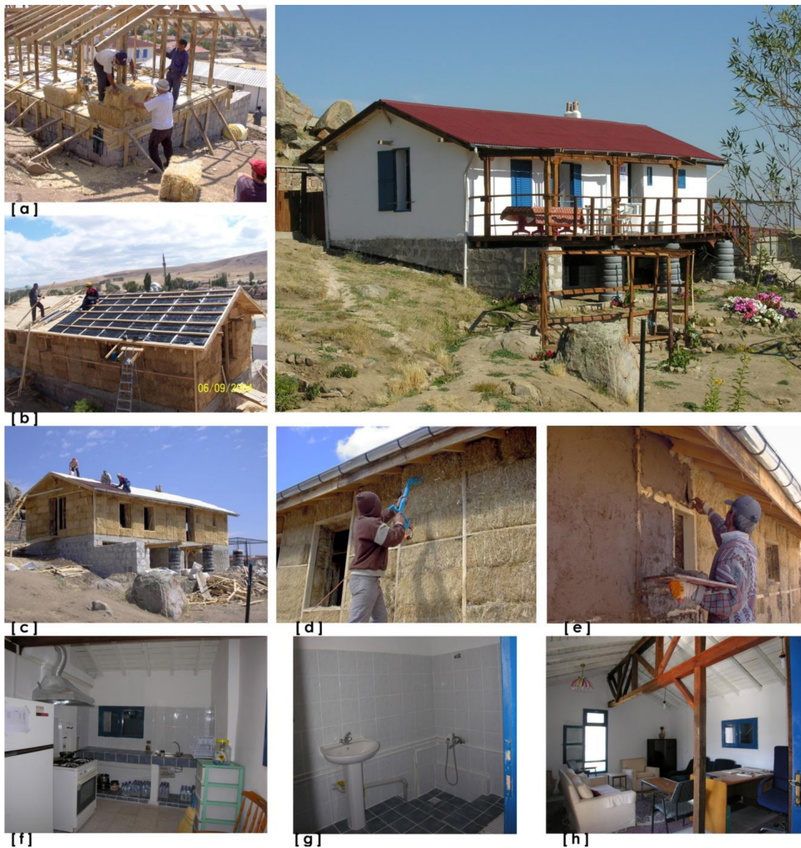
FIGURE 3. The Strawbale House: [a] Timber structure on stone foundations; [b] erecting the roof structure; [c] finishing the roof; [d] trimming the straw; [e] applying mud-plaster on the walls. [f] The kitchen; [g] bathroom; [h] and interior of the strawbale house.
