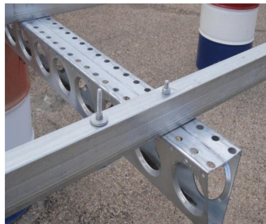
FIGURE 5. Set the rails.
