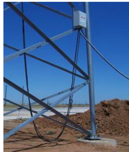
FIGURE 17. Tower junction box.
