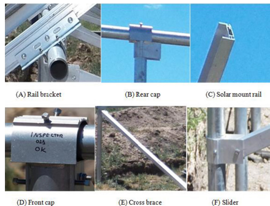
FIGURE 9. Six parts of fixed frame.
