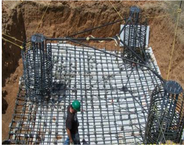
FIGURE 14. Bolt placement fixture with triangulated frame.
