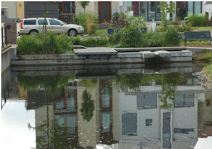
FIGURE 10. The stormwater areas are small but numerous. They treat small inflows and release them to another conveyance segment or into the saltwater canal as illustrated here. Recirculating the stormwater allows for multiple treatment opportunities. Photo by author, 2012.
