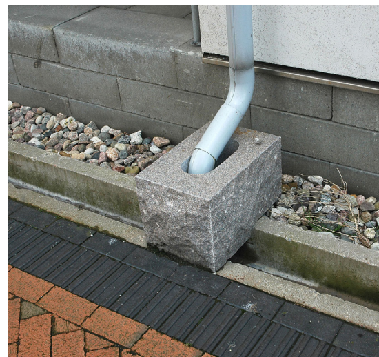
FIGURE 8. The infrastructure is exposed rather than hidden from the residents. The granite blocks and corrugated edging prevent accidents by increasing visibility. Photo by author, 2012.
