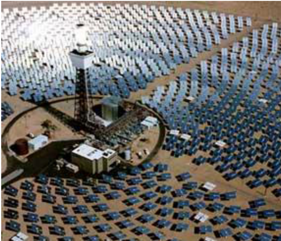
FIGURE 7. Power Tower systems, heliocentric mirrors focus on the tower and super hot transfer fluids then power a steam plant at the bottom of the tower. [13]
