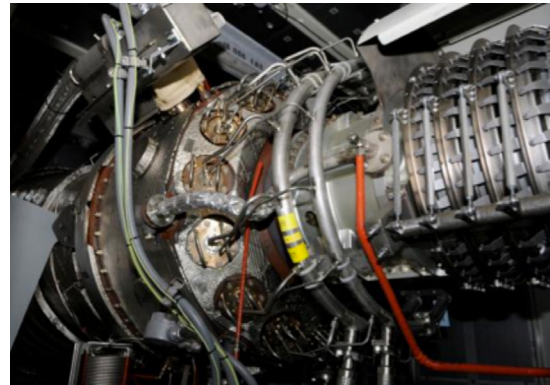
FIGURE 6. Gas turbine at the heart of the University of Calgary's cogeneration system.
