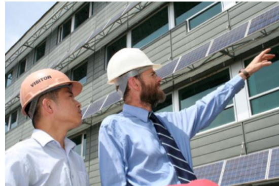
FIGURE 8. The Child Development Centre, note building integrated photovoltaic sunshades on south facade.
