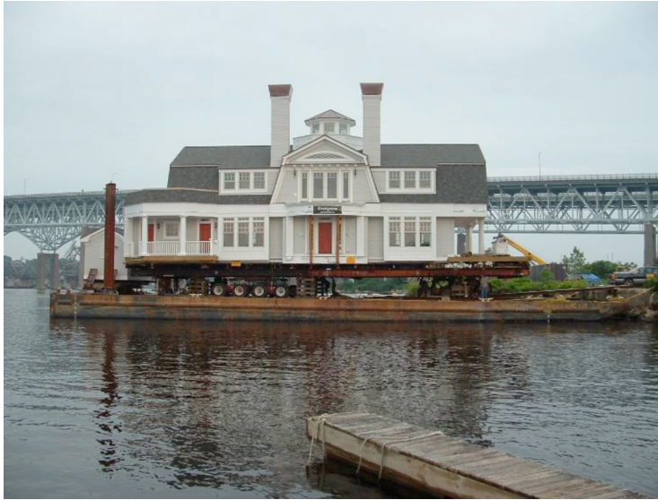
FIGURE 4. Put on barge in New London and shipped 75 miles west to Sumac Island.
