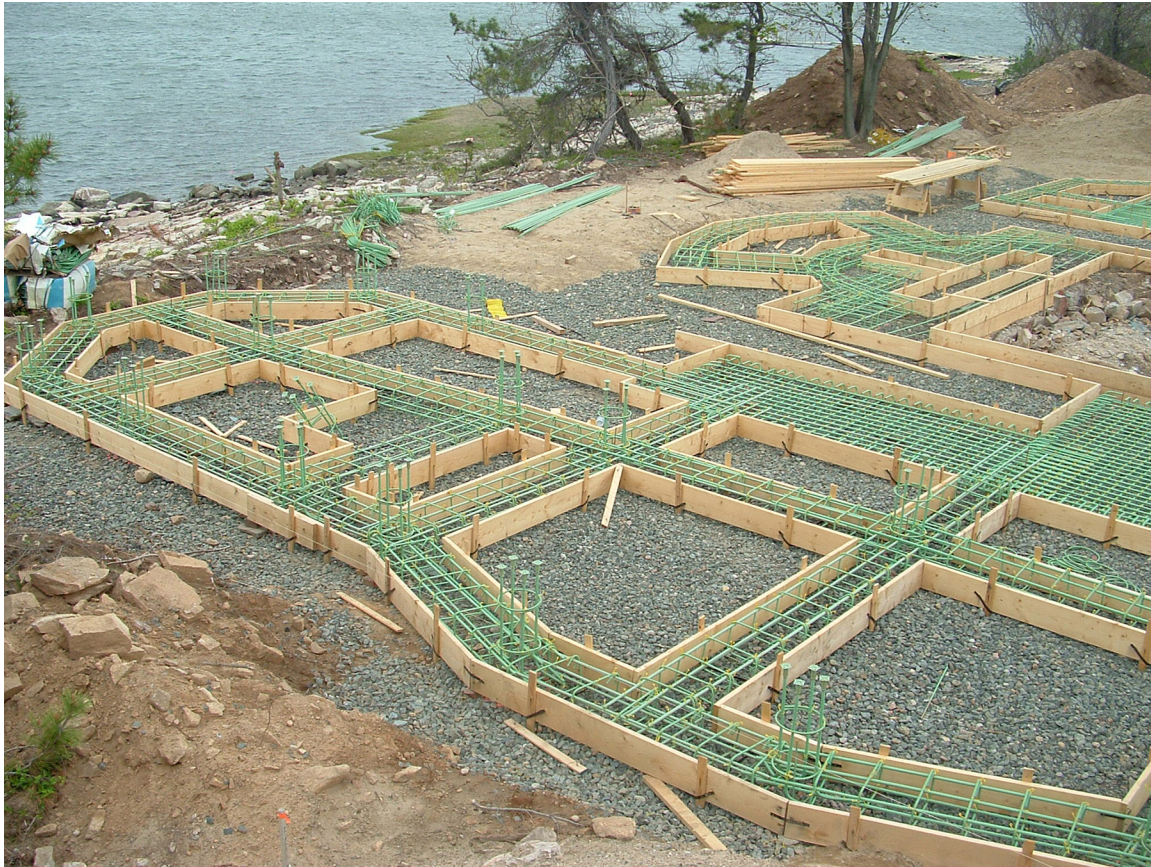
FIGURE 5. Mat Foundation.
