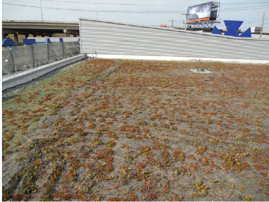
FIGURE 5. Lightweight extensive vegetated roof at the International Alliance of Theatrical Stage Employees Local 8 headquarters 10 months after installation . . . becoming established. (Courtesy Roofmeadow)
