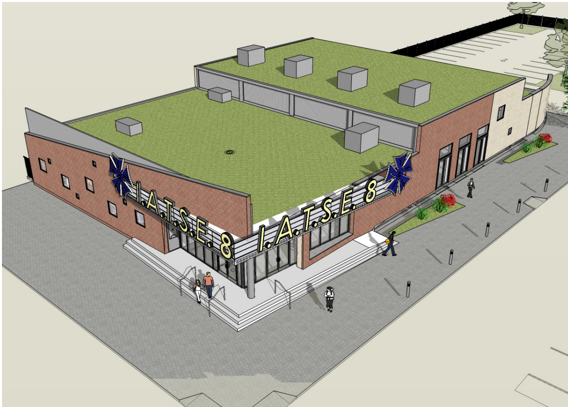
FIGURE 4. The International Alliance of Theatrical Stage Employees Local 8 headquarters has a 0.22 acre lightweight extensive vegetated roof. (Courtesy SaylorGregg)
