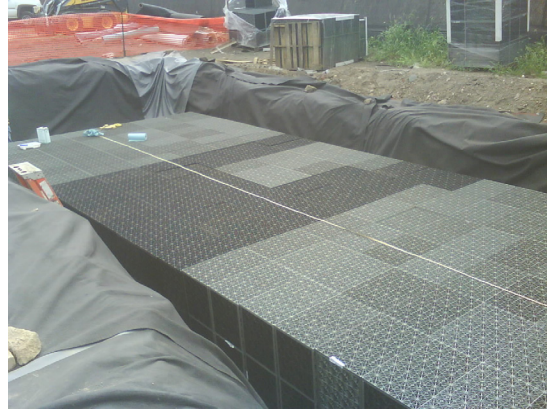
FIGURE 6. Subsurface rain tank detention system during installation prior to wrapping at the International Alliance of Theatrical Stage Employees Local 8 headquarters. (Courtesy SaylorGregg)
