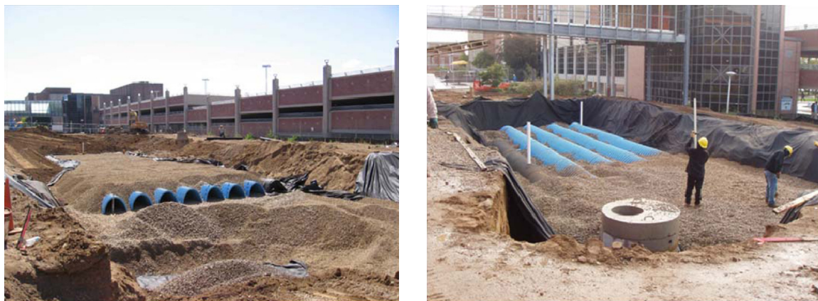
FIGURE 2. Examples of space constraints when installing stormwater retrofits at Western Michigan University, Kalamazoo, Michigan.
