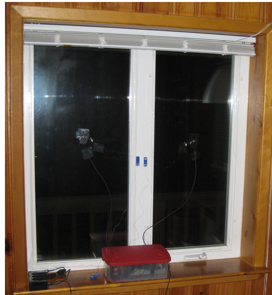
FIGURE 11. Interior plastic film on a case study window.
