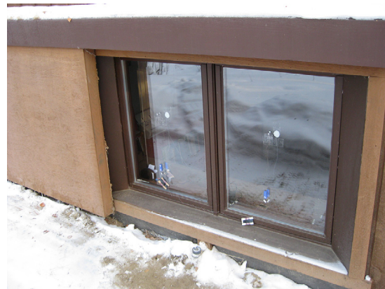
FIGURE 7. Exterior foam shutter system.
