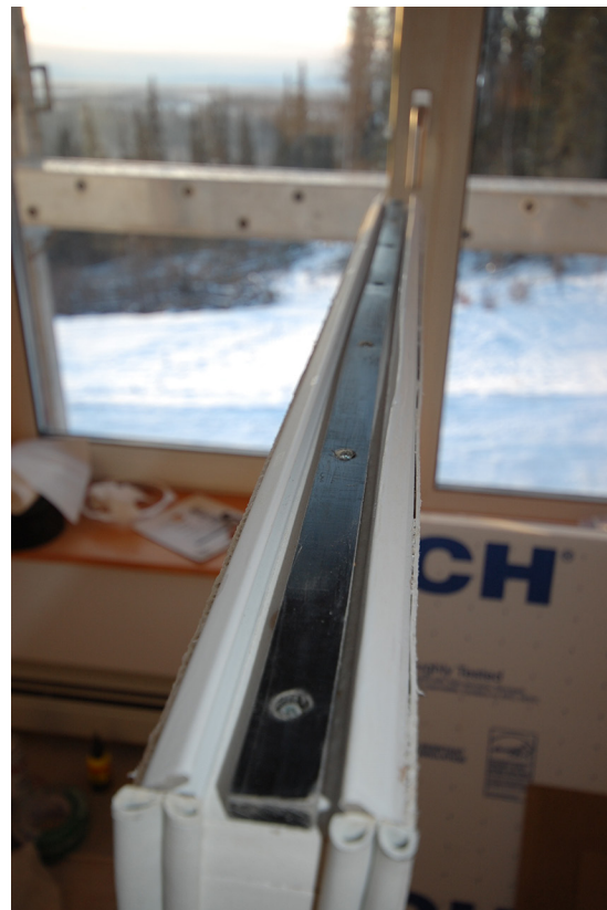
FIGURE 12. This interior shutter has weatherstripping to seal the window sill.
