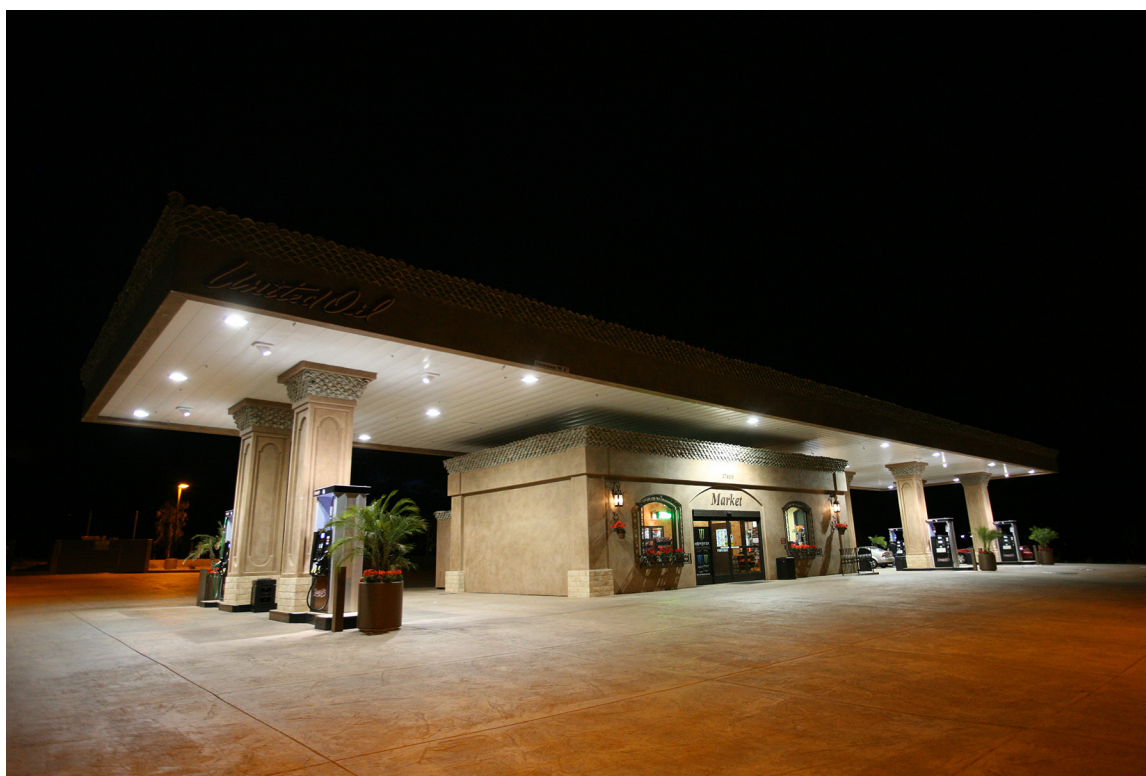
FIGURE 7. Dark-sky friendly lighting at a service station produces minimal glare, no up light, and uniform lighting with smooth transitions that the eye can easily adapt to.
