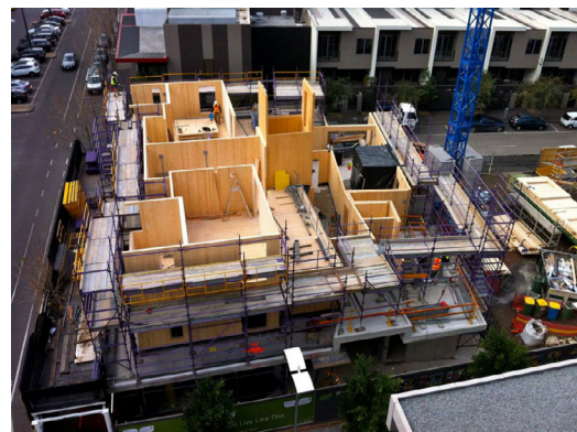
FIGURE 3. The 'Forte' building in Melbourne Docklands under construction, in July 2012. The 10-storey residential tower with 23 apartments is entirely prefabricated, using an engineered solid wood panel construction system; the building stores around 1,400 tonnes CO 2 in its structure (Photos: the author, July 2012).
