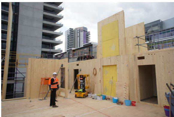
FIGURE 3. The 'Forte' building in Melbourne Docklands under construction, in July 2012. The 10-storey residential tower with 23 apartments is entirely prefabricated, using an engineered solid wood panel construction system; the building stores around 1,400 tonnes CO 2 in its structure (Photos: the author, July 2012).
