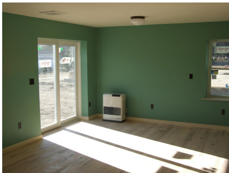
FIGURE 6. With the excellent envelope, this gas heater can provide space heating to the entire home.
