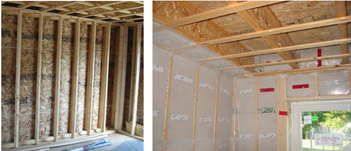
FIGURE 5. Double walls before and after cellulose insulation.
