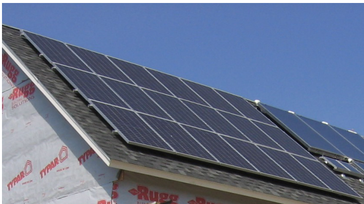
FIGURE 9. Solar collectors installed on one home during construction. Solar electric modules (PV) are on the left; solar thermal collectors are in the background to the right.
