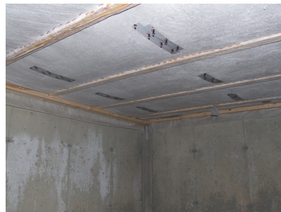
FIGURE 3. Ceiling of a basement insulated with blown cellulose.
