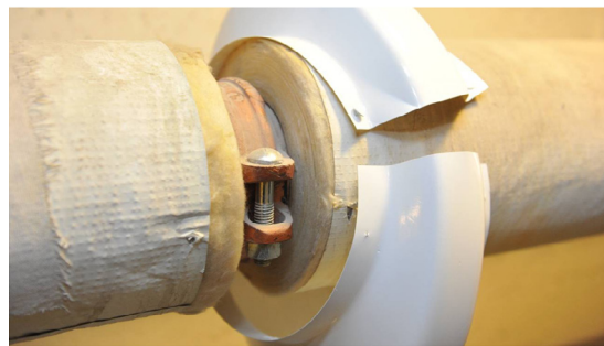
FIGURE 3. Sweating pipes with improper insulation and insufficient spacing in a medical building.
