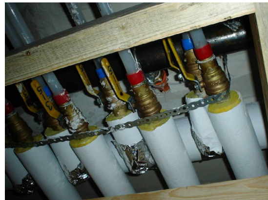
FIGURE 5. Example of Building 2 Modeled Condition : New domestic hot water pipes (risers) before drywall application—poor practice and material choice.
