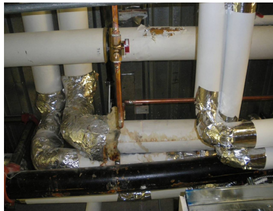
FIGURE 3. Sweating pipes with improper insulation and insufficient spacing in a medical building.
