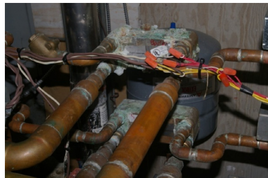
FIGURE 4. Example of Building 1 Modeled Condition : Detail showing heat exchangers used with domestic water system. Note the build up of deposits on the heat exchangers.
