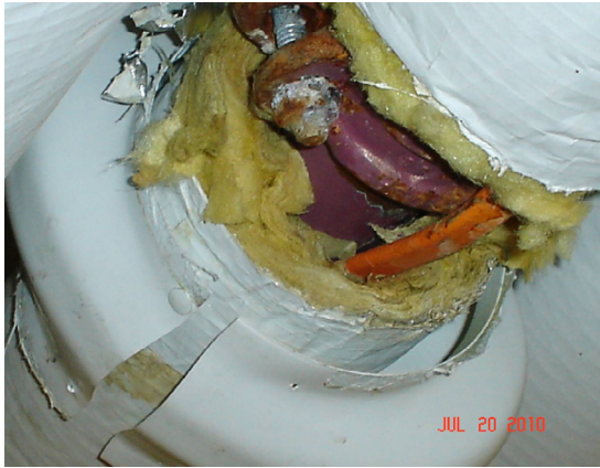
FIGURE 1. Corrosion and condensation in new LEED Platinum multi-family residential building.
