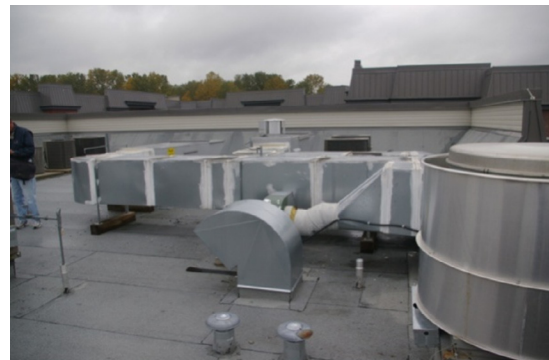
FIGURE 7. Example of Building 3 Modeled Condition : A section of an un-insulated supply air duct on a roof mounted make-up air unit.
