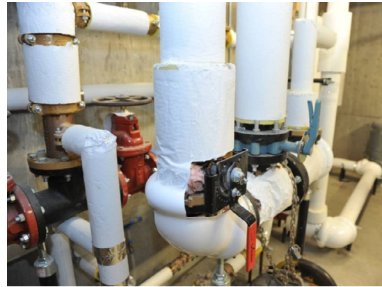
FIGURE 6. Example of Building 2 Modeled Condition : New mechanical room—poor practice and material choice.
