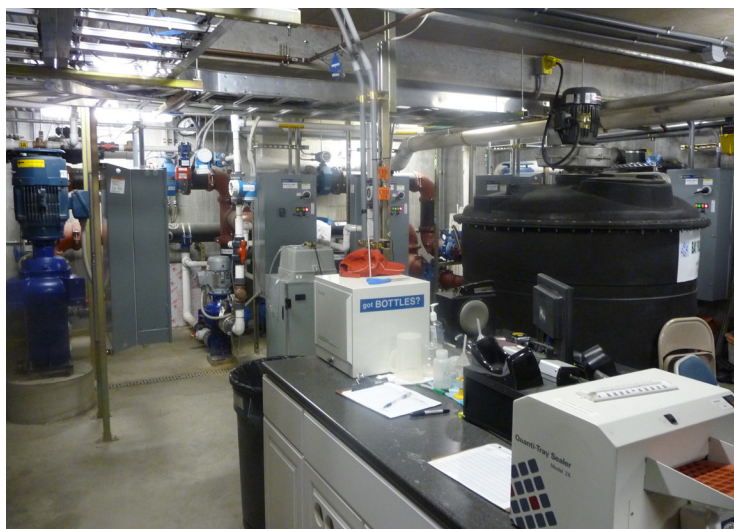
FIGURE 8. The membrane bioreactor (MBR) system situated in the basement of the OHSU CHH building treats up to 30,000 gallons of waste water per day, providing a source of reclaimed water for toilet flushing and other non-potable uses throughout the building, and enabling the building to use no potable water for toilet flushing.
