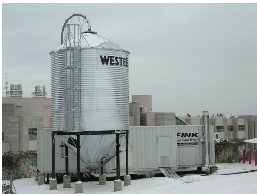
FIGURE 3. Left: Wood pellet heating system for the Enhanced Forestry Laboratory. The fuel silo feeds pellets into the shipping container where a boiler heats water for the building. An emissions filtration system results in particulate emissions that are below natural gas levels. Right: Doug Carter, project manager for the two bioenergy projects, with the wood pellets which are burned in the KOB boiler.
