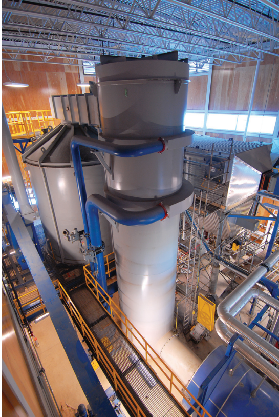
FIGURE 7. The interior of the Bioenergy Plant, showing the Nexterra gasifier (back left), oxidizer (centre), boiler (lower right), conveyor (bottom left), and electrostatic precipitator (right).
