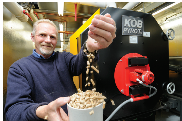
FIGURE 3. Left: Wood pellet heating system for the Enhanced Forestry Laboratory. The fuel silo feeds pellets into the shipping container where a boiler heats water for the building. An emissions filtration system results in particulate emissions that are below natural gas levels. Right: Doug Carter, project manager for the two bioenergy projects, with the wood pellets which are burned in the KOB boiler.
