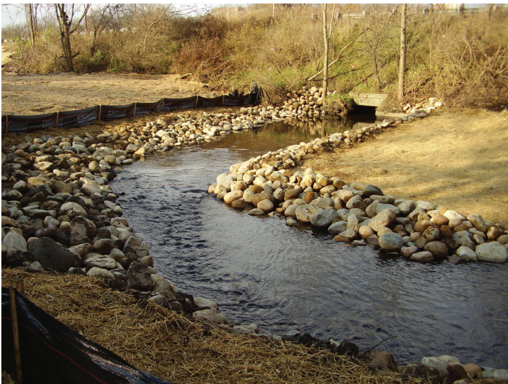
FIGURE 7. Streambank stabilization of previous erosion areas in Arcadia Creek along Stadium Drive, Kalamazoo, Michigan. (Substantial completion photograph, November, 2011.)
