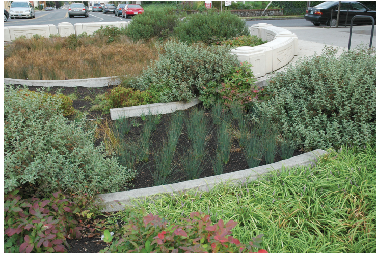
FIGURE 1. Bioretention for treating road runoff on Sandy Blvd. in Portland, Oregon (Austin, 2011).
