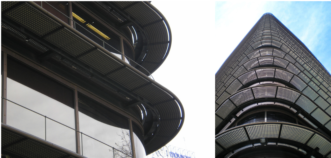
FIGURE 3. Banco de Bilbao, Madrid, 2008, Corner Marquesina and solar protection details, photographer: César Martín Gómez.
