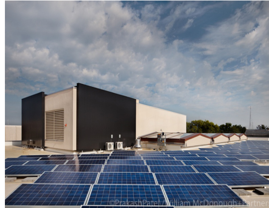
FIGURE 3. Solar PVs and Solar Transpiration.
