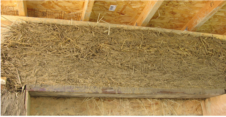
FIGURE 3. Un-plastered straw light clay above a lintel.
