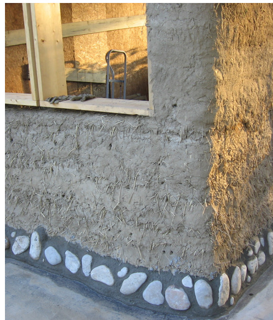
FIGURE 2. Un-plastered cob wall with fieldstone used to cover an on-grade 'earthbag' foundation.
