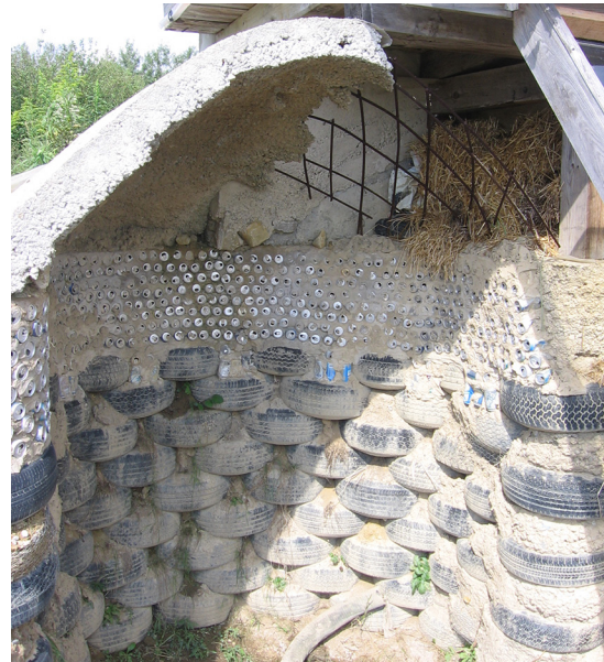
FIGURE 1. Rammed earth tires. The pop-can wall comes from Michael Reynold's 'Earthship' design.
