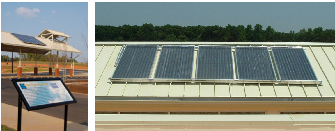
FIGURE 7. Photovoltaic and Solar Hot Water Heating Systems.
