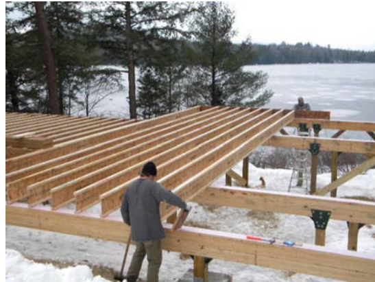
Base frame with continuous joists being placed.
