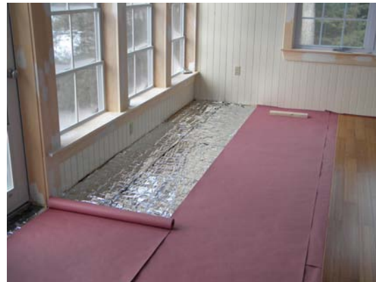
Radiant barrier under 3-season room floor.
