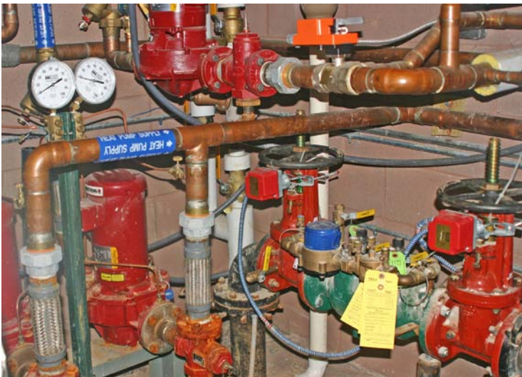
FIGURE 7. Geothermal HVAC system pipes and pumps (with valves to fire sprinkler system).
