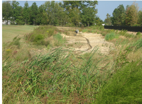
FIGURE 3. Extended Detention Basin.
