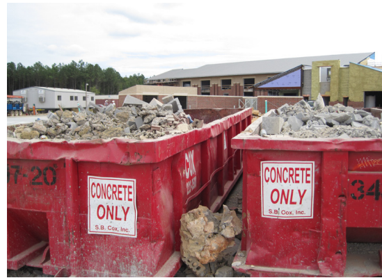
FIGURE 7. Construction Waste Recycling.
