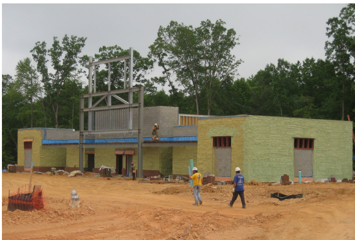
FIGURE 4. Air Barrier on Field House.
