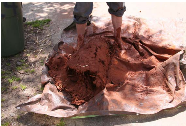
FIGURE 1. Mixing cob using the tarp method.
