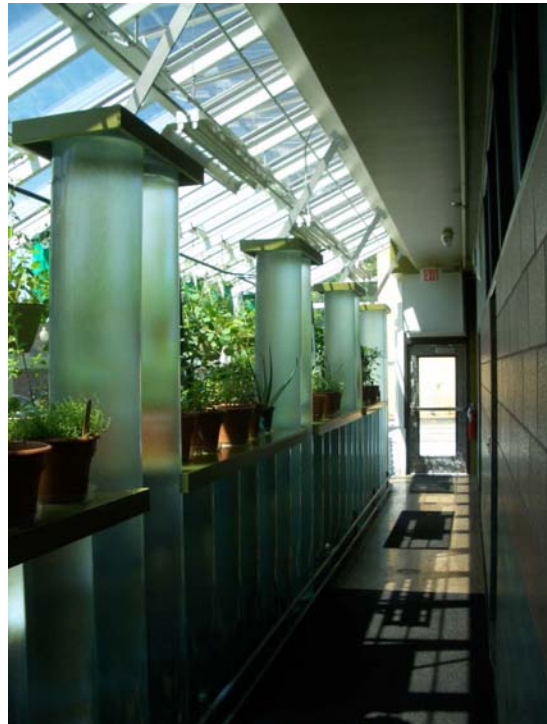
FIGURE 18. View of New Water Tube Thermal Mass Wall at New Greenhouse Corridor.
