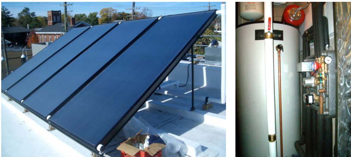
FIGURE 9. Solar Domestic Hot Water Collectors (4 Panels) and Solar Pre-Heat Tank.
