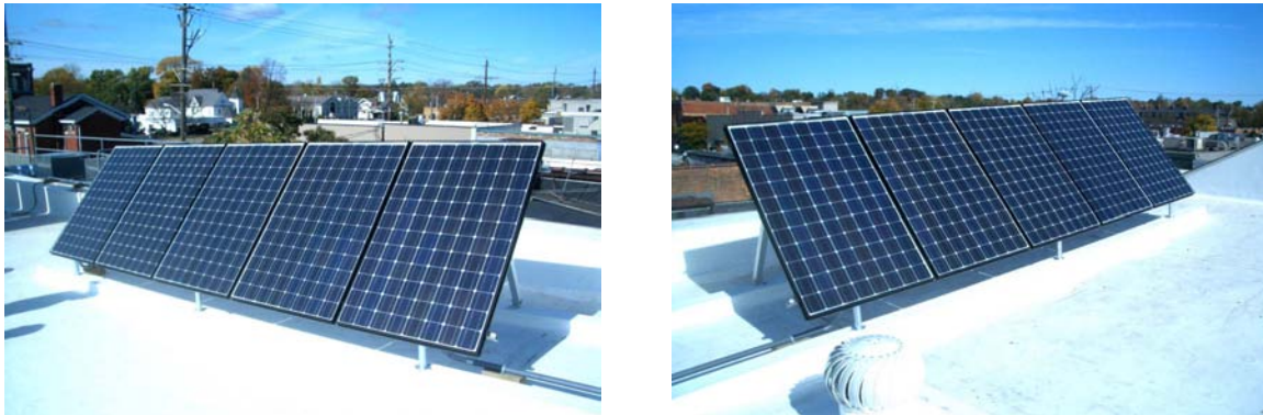
FIGURE 8. G.E. Photovoltaic Solar Electric Panels (2 Banks of 5 Panels @ 250 W / Panel).
