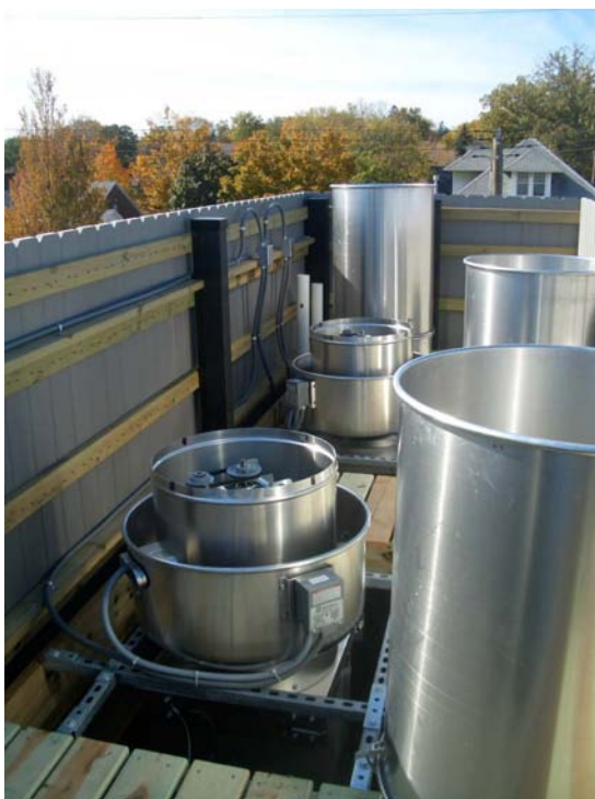
FIGURE 6. Variable Air Volume Rooftop Exhaust Fans (2) and 14’ Kitchen Hood.
