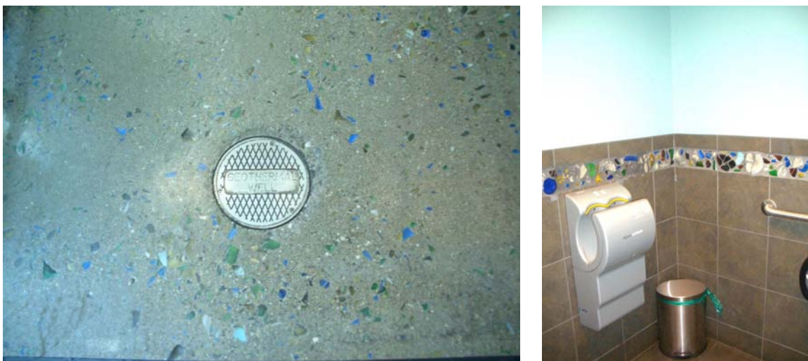
FIGURE 15. Recycled Colored Glass Aggregate for Conc. Floors and Wall Feature Strips.
