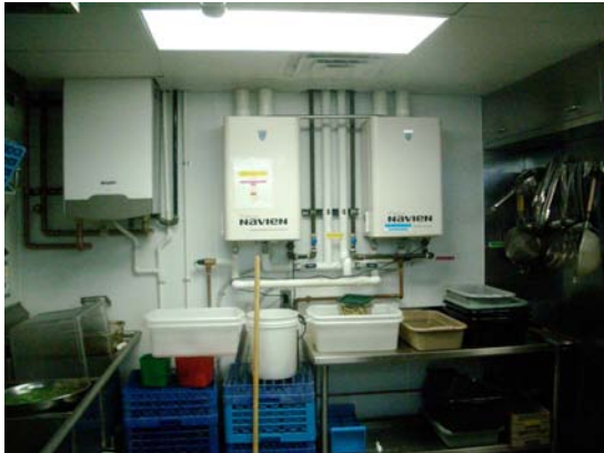
FIGURE 4. Instantaneous Gas Fired Boilers and Electric Fired Water Heaters.
