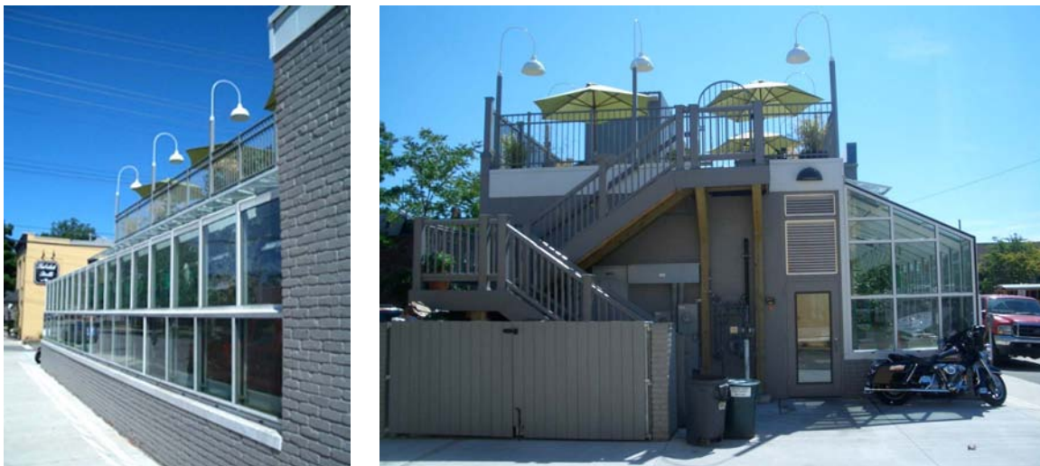
FIGURE 16. Recycled Brick Veneer for New Addition and Trash Enclosure Exterior Walls.
