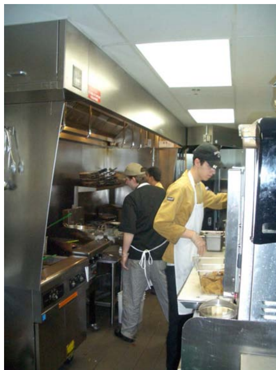
FIGURE 6. Variable Air Volume Rooftop Exhaust Fans (2) and 14’ Kitchen Hood.
