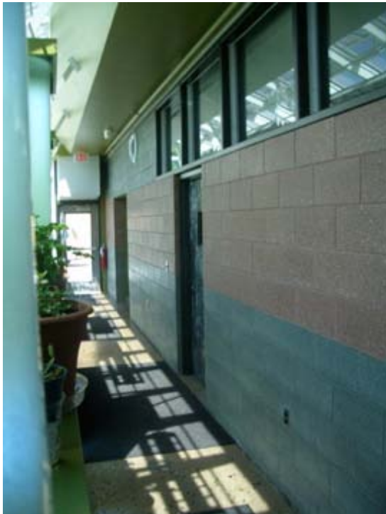
FIGURE 17. View of New CMU Trombe Thermal Mass Wall at New Greenhouse Corridor.
