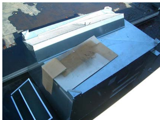
FIGURE 5. Rooftop Energy Recovery Ventilator (ERV).
