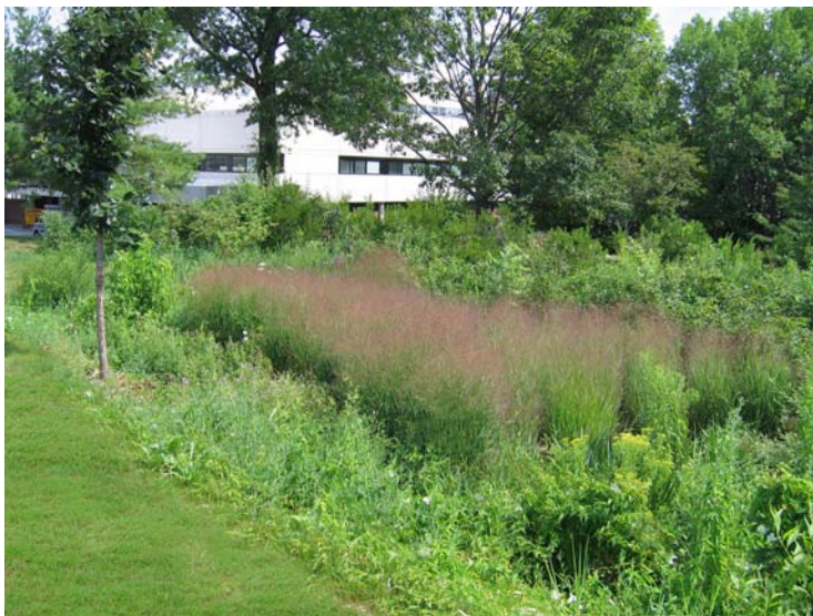
FIGURE 3. The bioretention basin holds and filters stormwater from parking areas.
