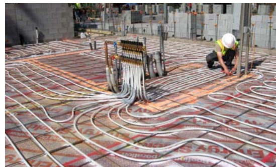
PEX in-floor cooling/heating loops being installed.
