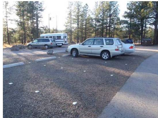
Parking spaces paved in pervious GravelPave® system.
