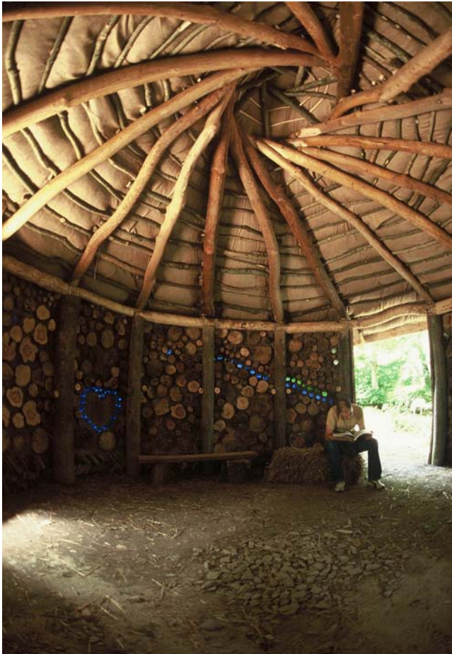
FIGURE 7. Round house built with round wood.
