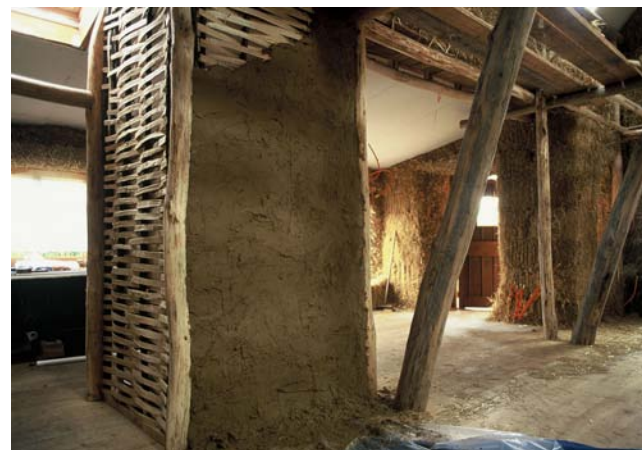
FIGURE 4. Wattle and daub on roundwood timber frame. Woodsman's home in East Sussex.
