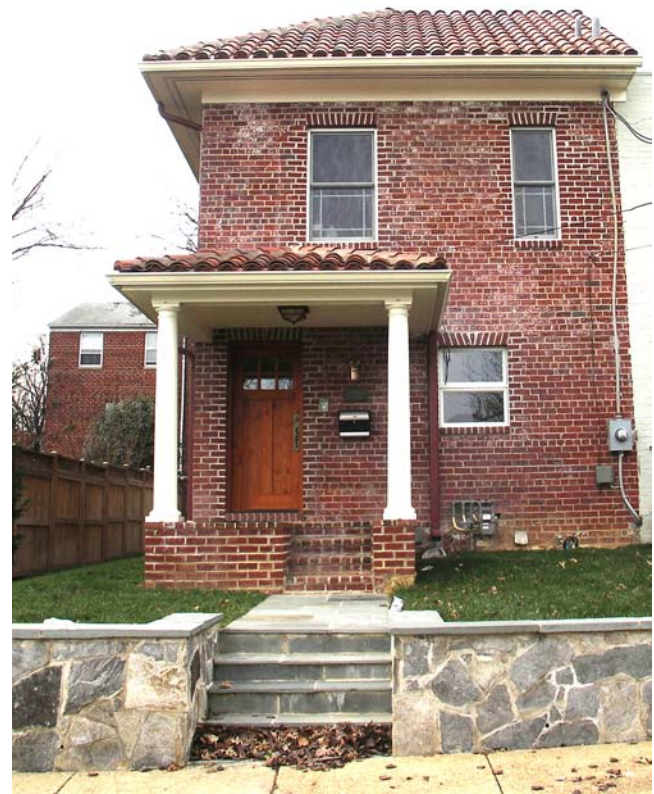
FIGURE 13. Exterior photograph of front elevation showing new porch, new taller windows (with the exception of the kitchen window), and the new roof. Photograph was taken during construction.
