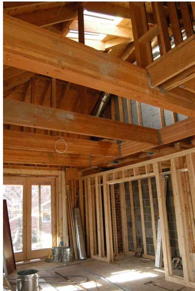
FIGURE 10. Interior construction photo showing patio doors on first floor, exposed beams in 2-story Master Bedroom, and opening for skylights above.
