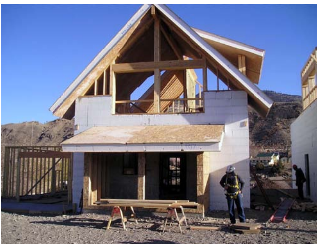
FIGURE 6. ICF wall construction and SIP roof construction. (Photo: Erik Hendrickson)
