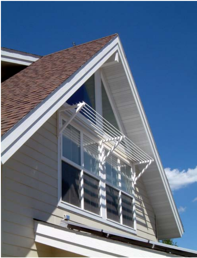
FIGURE 9. South windows showing shading at summer midday. (Photo: A. Denzer)
