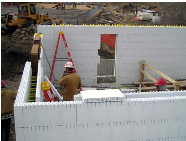
FIGURE 5. ICF wall construction. (Photo: Erik Hendrickson)
