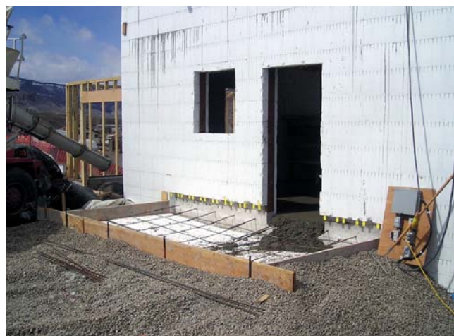
FIGURE 10. Sunspace construction. Note slab thickness at left, removal of wall insulation at right. (Photos: Erik Hendrickson)
