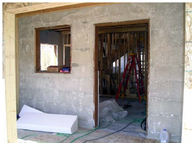
FIGURE 10. Sunspace construction. Note slab thickness at left, removal of wall insulation at right. (Photos: Erik Hendrickson)
