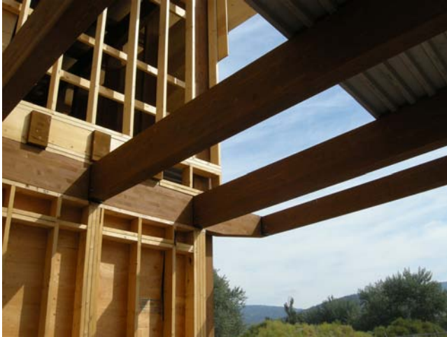
FIGURE 8. Timber-framed construction.
