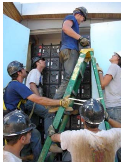
Project Solar House—under construction in Manhattan, Kansas (structural insulation panels and battery bank).
