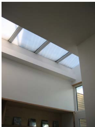
Bedroom skylight. The skylight is filled with translucent insulation, allowing light through while minimizing heat transfer. The shadow on the aperture is cast by the solar hot water system, further diminishing heat gain.
