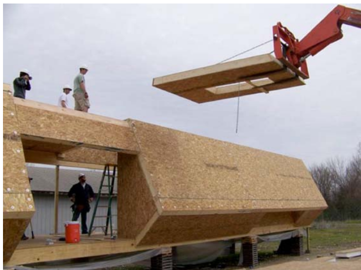
Project Solar House—under construction in Manhattan, Kansas (structural insulation panels and battery bank).
