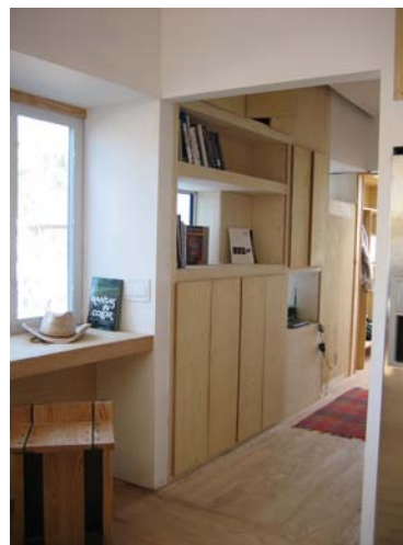
Hallway. The north façade of the hall and bedroom (beyond) were made a storage wall, built around the translucent north apertures. This heightens the separation between the exterior of the building and these private spaces. Most of the building's electronics are housed in the cabinets here.
