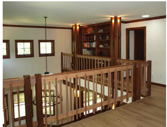
Interior trim and finishes using inexpensive (#2 cedar) or reclaimed lumber.
