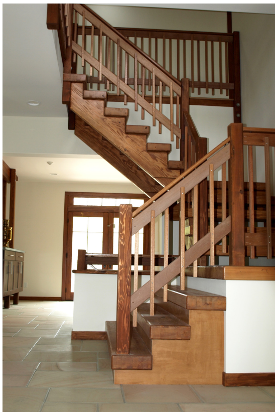
Stair built from reclaimed glue lams.
