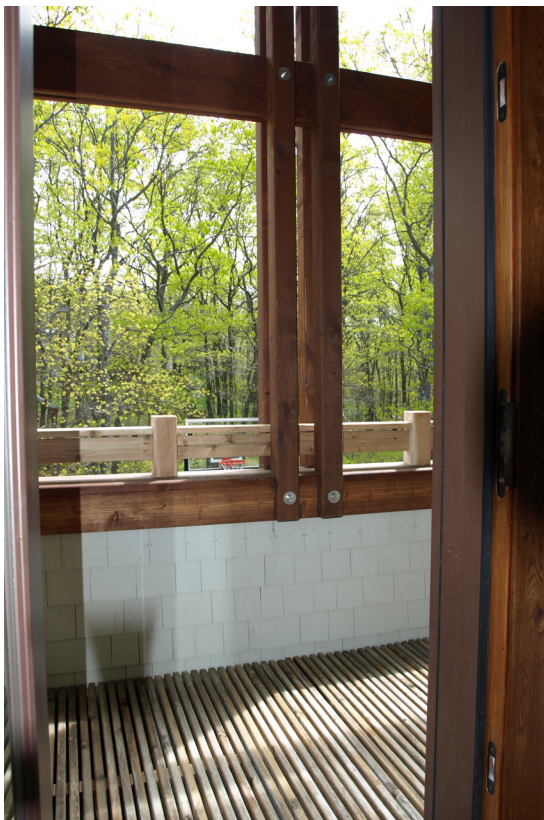
5/4 decking sliced in half for edge exposed decking.
