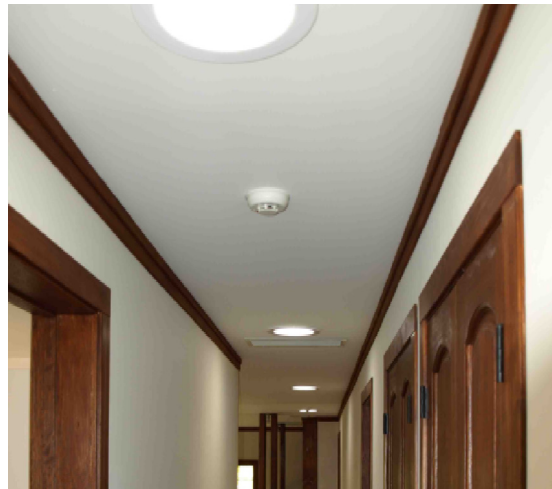
Sola-Tubes light the second-floor hallway.
