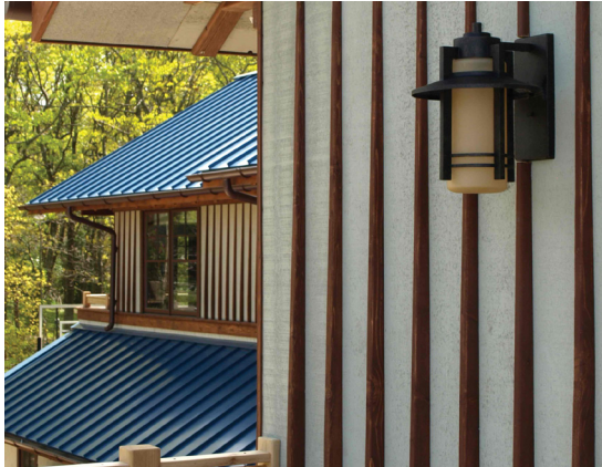
Re-claimed siding re-cut and used for trim.
