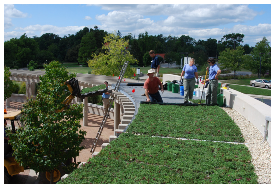
FIGURE 2. Installing ballast and green roof modules on west arbor arm, Minnetrista, September 2008. Photo credit: Minnetrista.
