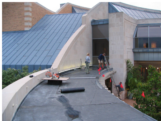
FIGURE 1. Installing waterproofing membrane and flashing on west arbor arm for Minnetrista green roof, September 2008. Photo credit: Minnetrista.
