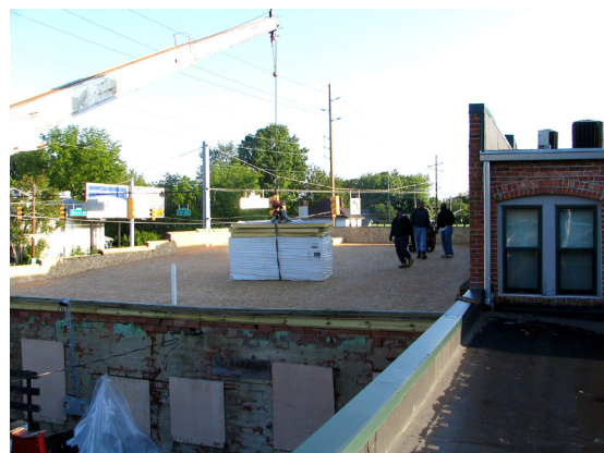
FIGURE 3. Replacement of roof deck, Moonblock Building, May 2007. Photo credit: John H. Boner Community Center.
