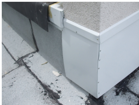
FIGURE 12. 3Mass waterproofing installation: bitumen membrane carried up parapet wall, with extra layer of EPDM before finishing with coping. April 2009. Photo credit: AAA Roofing.
