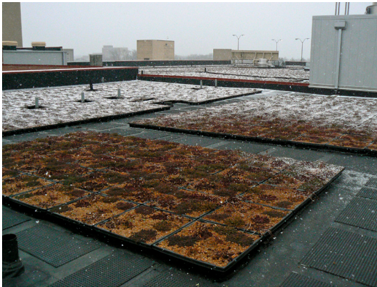
FIGURE 11. BMH green roof and walkways, January 2010. Areas not covered by snow are located near heat vents. Photo credit: Anne Altor.
