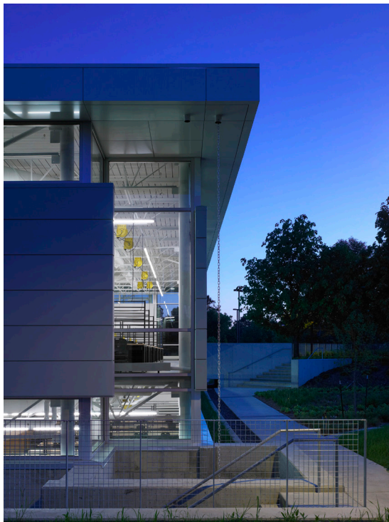
FIGURE 10. This image shows the rain chain on the northeast corner of the building—water moves from the green roof down the rain chain into the concrete detention cell that is part of the site’s stormwater management system.
