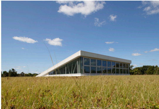
FIGURE 7. This photograph was taken on the green roof, and shows the sloped roof monitor emerging from the vegetated roof. The windows are operated by a control system with which the students and faculty can interact.
