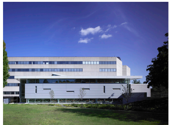
FIGURE 6. This image shows the recessed profile of the addition with the existing college of design facility in the background. Notable features: clerestory window bands, small operable windows for views from classrooms as well as natural ventilation. Rooftop light monitor is also apparent.
