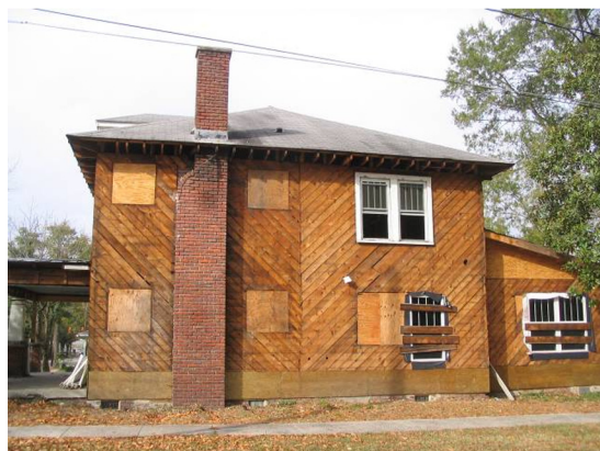
FIGURE 1. The sheathing on an old home can have up to seven times the penetrations, and the wood materials tend to be less uniform than new wood, leading to increased air infiltration. Some old homes lack any sheathing, where siding is tacked directly to studs.
