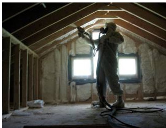
FIGURE 8. Spray foam insulation fully fills the stud cavities, simultaneously insulating and air sealing.
